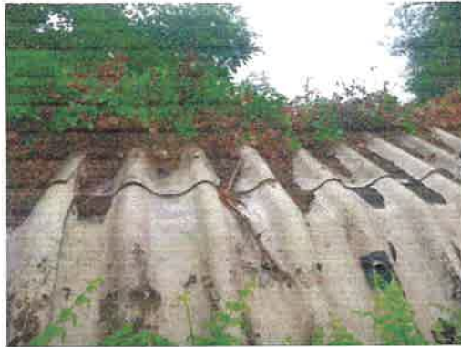
Photograph 5. Concrete asbestos roof (side elevation).
