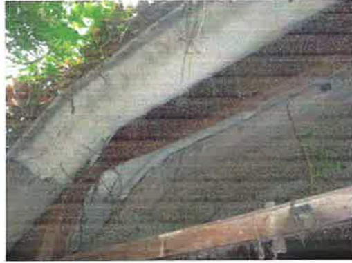
Photograph 6. Large hole above door frame (front elevation).
