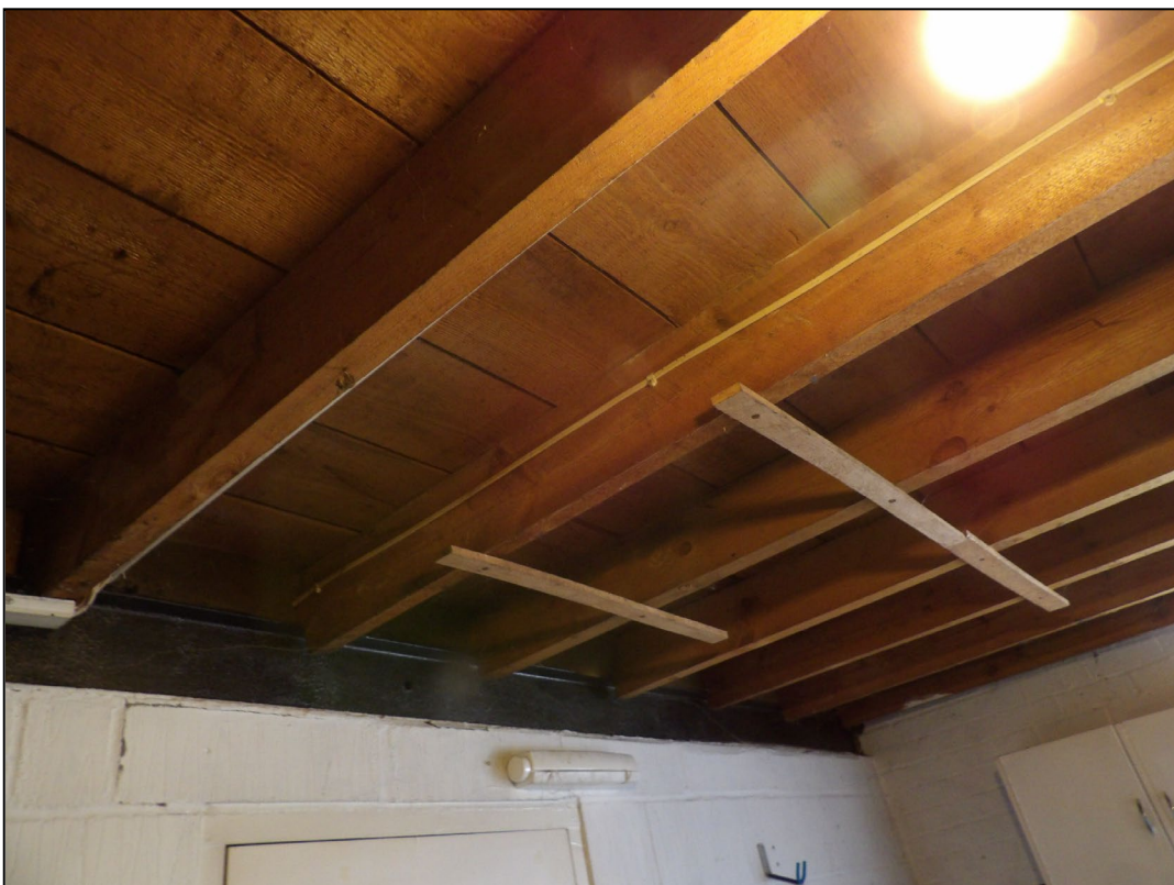
Figure 15. Limber lined ceiling of garages. 2 Ardwell Close, Crowthorne. 15.07.25
