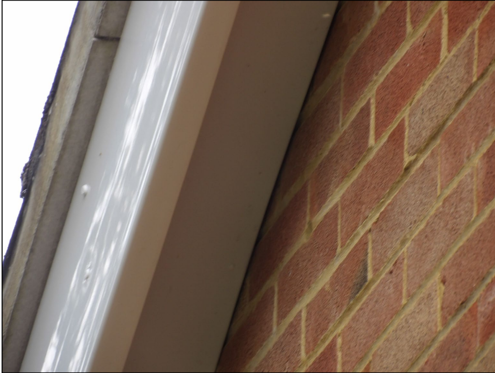
Figure 7. Example uPVC soffits and fascias. 2 Ardwell Close, Crowthorne. 15.07.25
