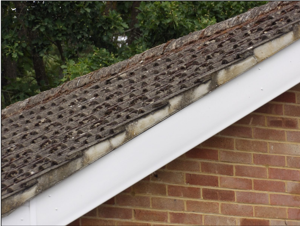
Figure 5. Example sealed verges. 2 Ardwell Close, Crowthorne. 15.07.25
