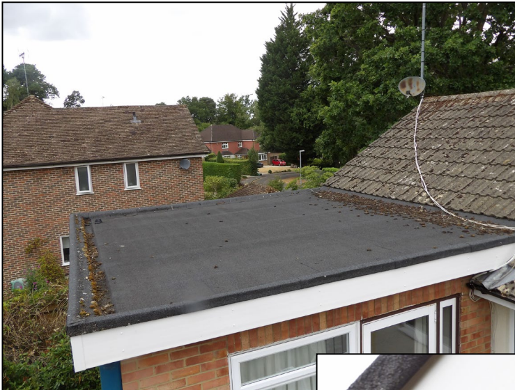
Figure 10. Roof and uPVC soffits/fascias on rear extension. 2 Ardwell Close, Crowthorne. 15.07.25
