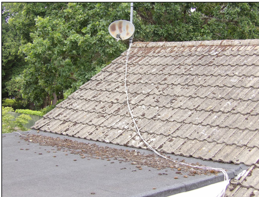
Figure 4. Tightly fitted roof and ridge tiles. 2 Ardwell Close, Crowthorne. 15.07.25
