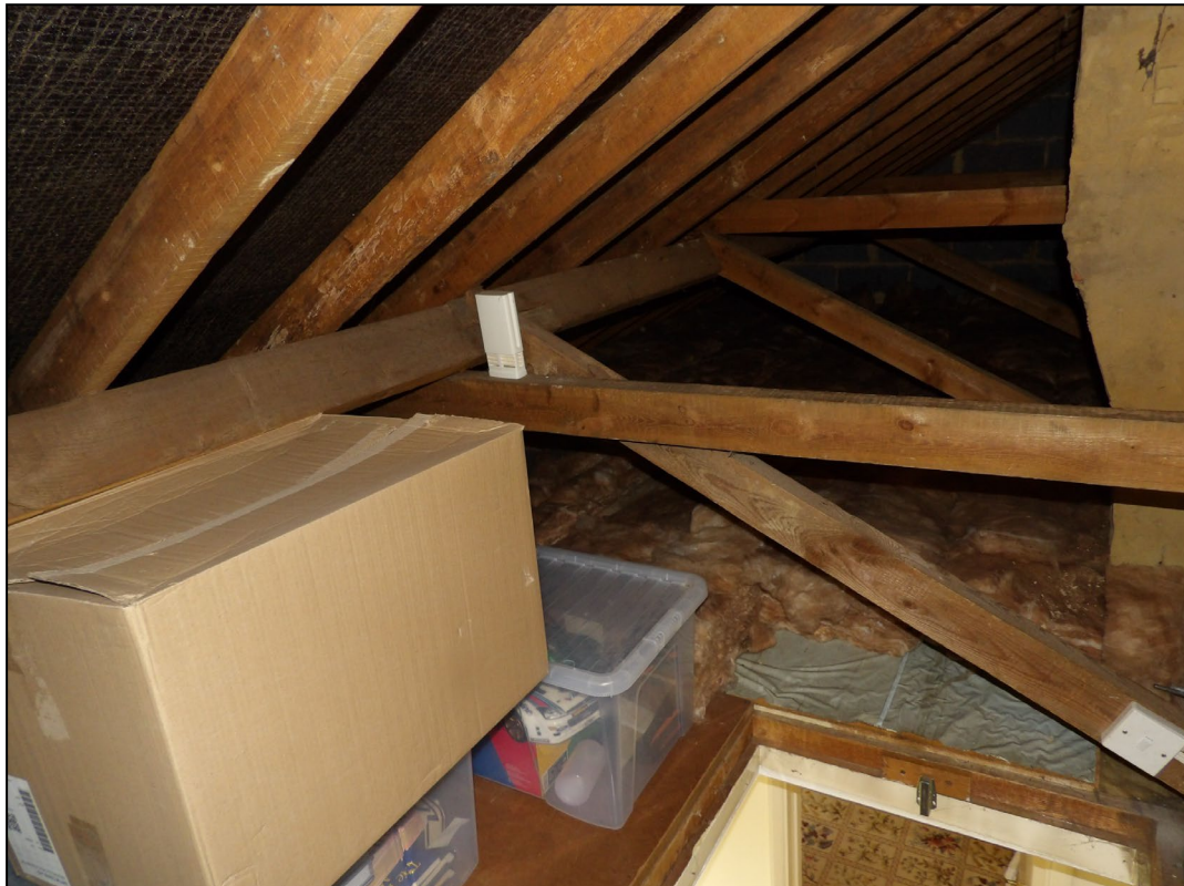
Figure 13. Example of loft space. 2 Ardwell Close, Crowthorne. 15.07.25
