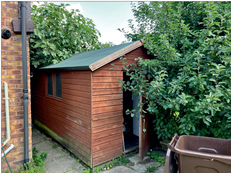
Photograph 4: Showing the timber shed within the garden area.
