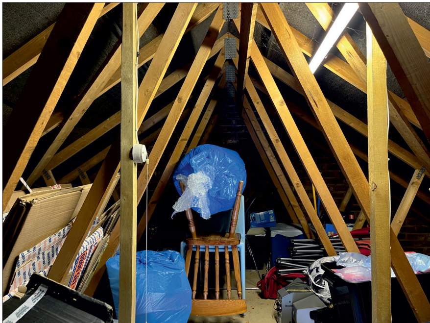
Photograph 3: Showing the roof space above the detached garage, which was cluttered with trusses.
