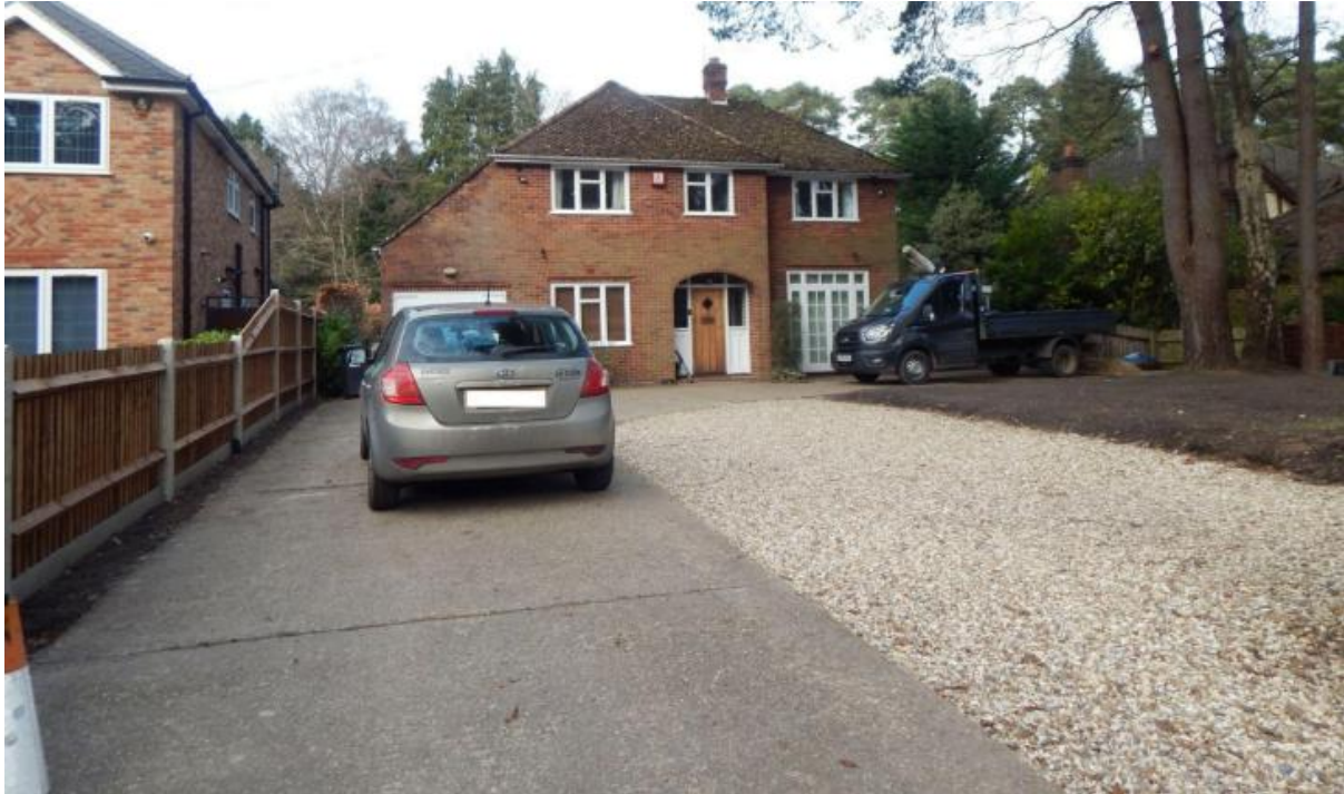
Image 1 – Front habitats of the site and South facing elevation of the property
