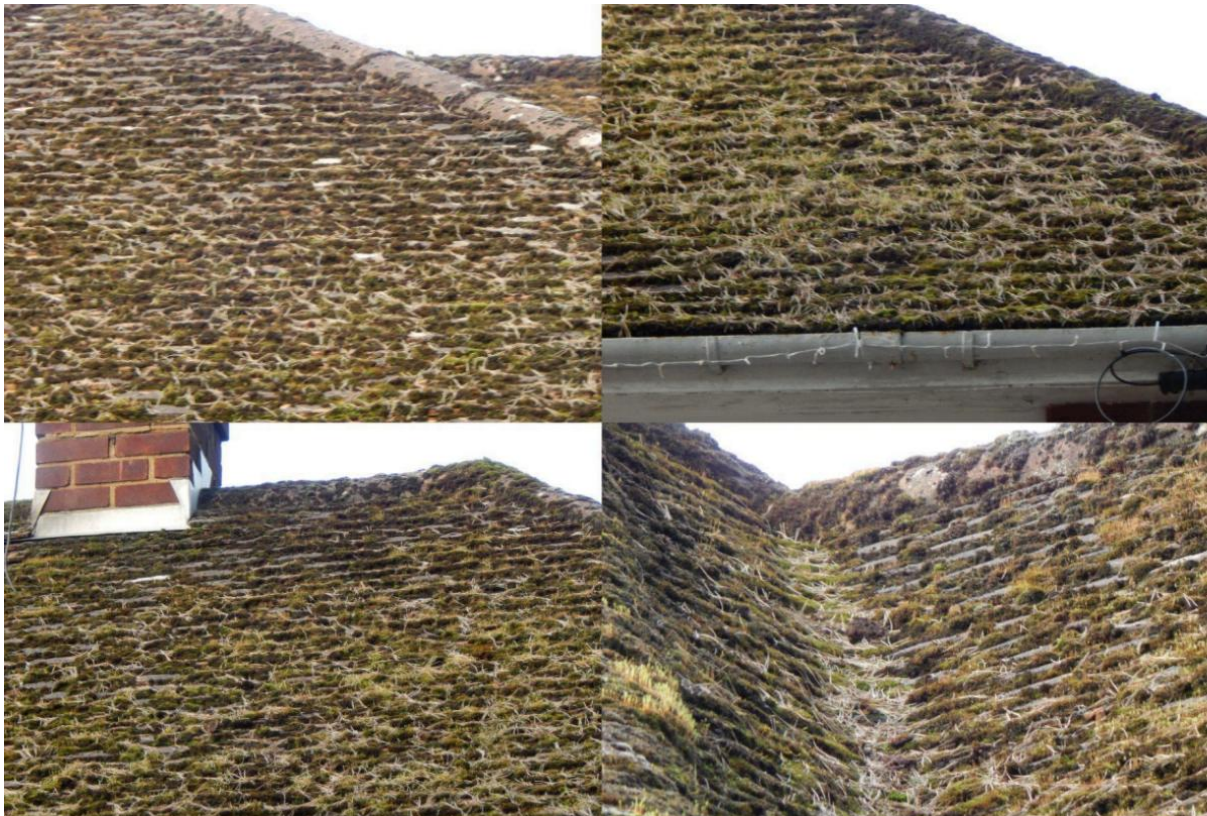
Image 2 – Front South facing roof coverings which offer a moderate covering from moss which may obstruct visibility of any suitable gaps of value to bats throughout
