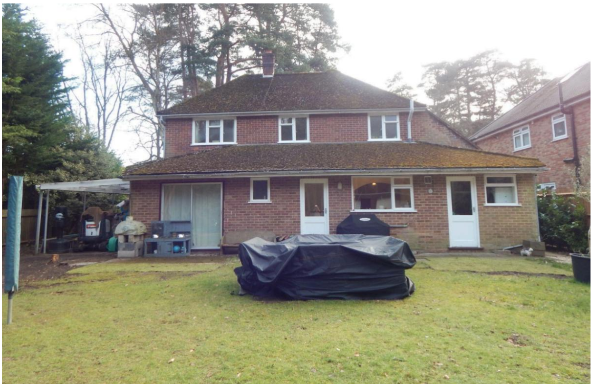
Image 4 – North facing elevation of the property
