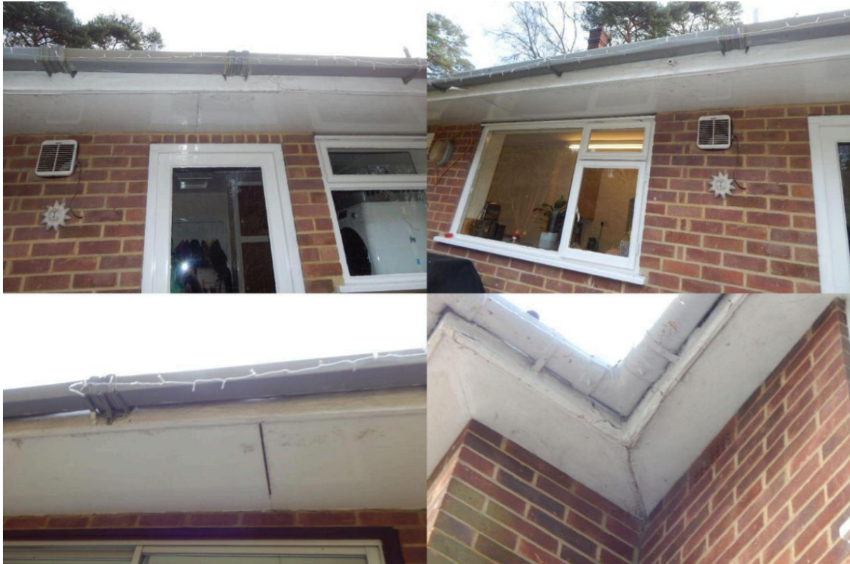
Image 7 – View of the main eaves coverings which have demonstrated a fair level of condition throughout
