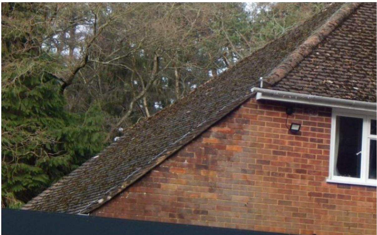
Image 6 – West facing elevation of the property
