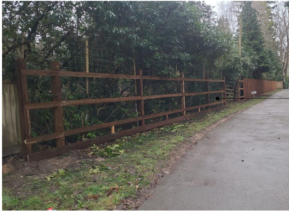
NEW FENCE STRUCTURE
