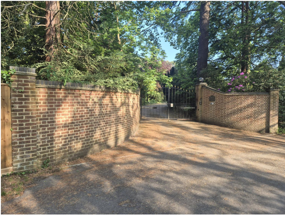
RETAINED ENTRANCE GATE
