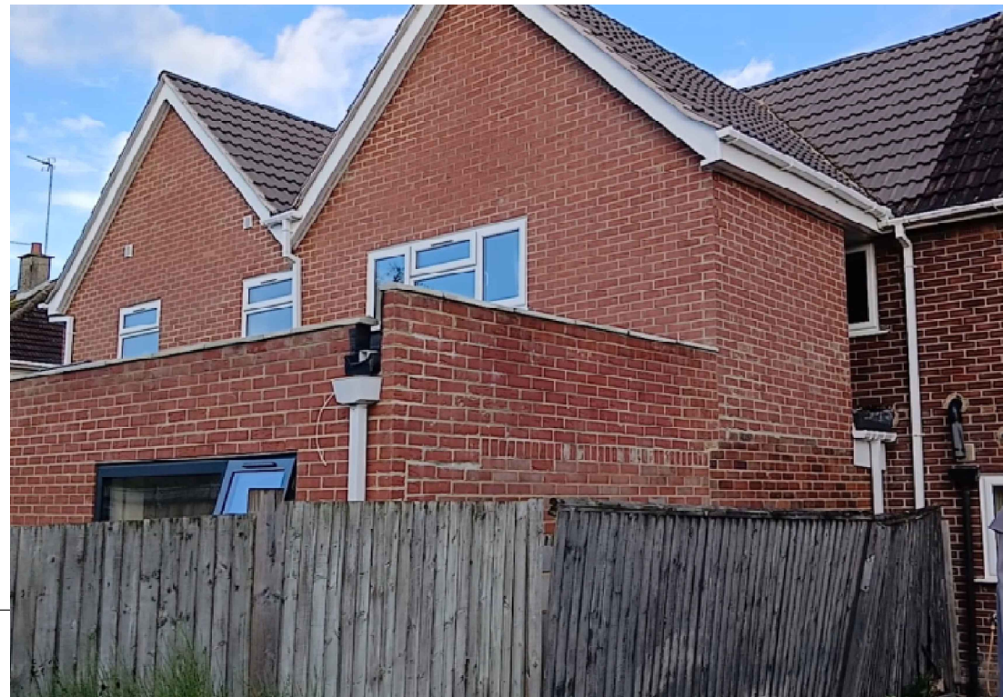
04 Photograph of Rear Extension to 91 Haddon Drive HDAA2 SCALE: N.T.S
