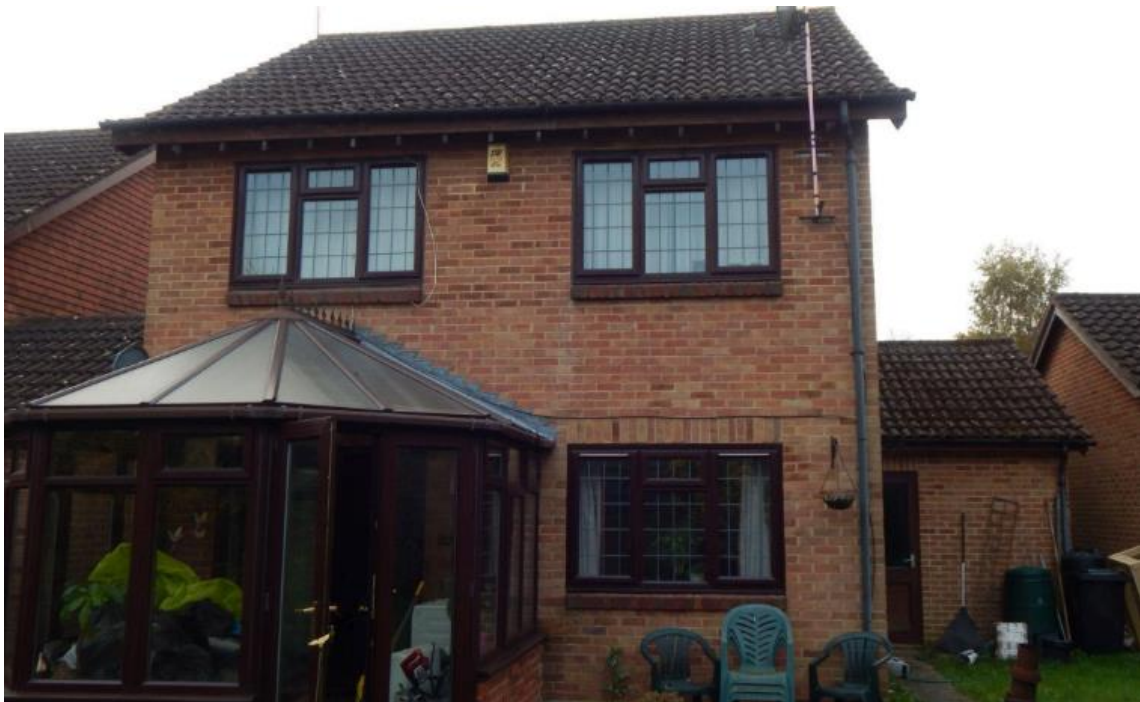
Image 4 – West facing elevation of the property
