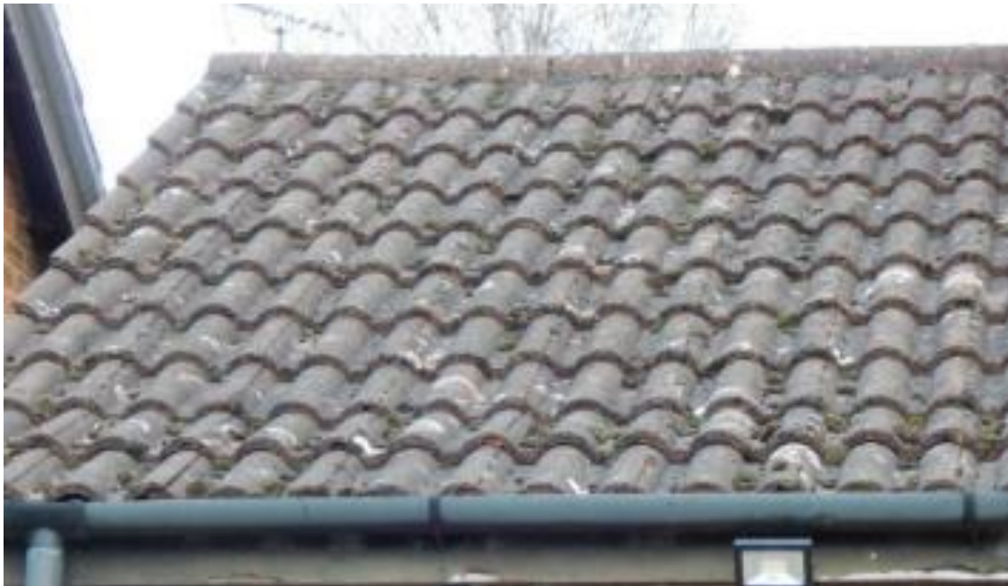
Image 2 – Close view of the lower West facing roof coverings to the property
