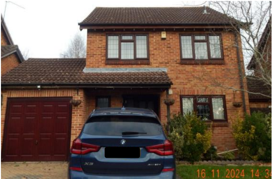
Image 1 – West facing elevation of the property
