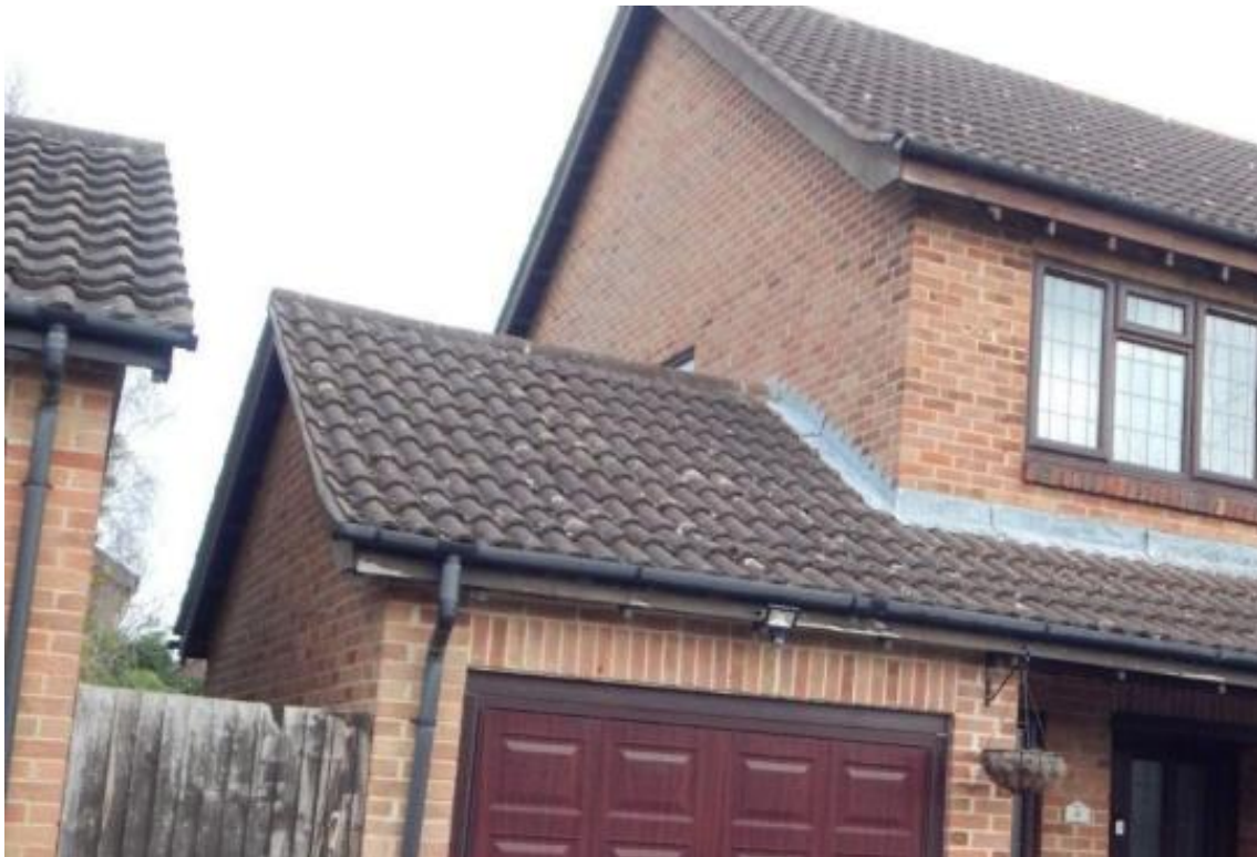
Image 6 – North facing elevation of the property
