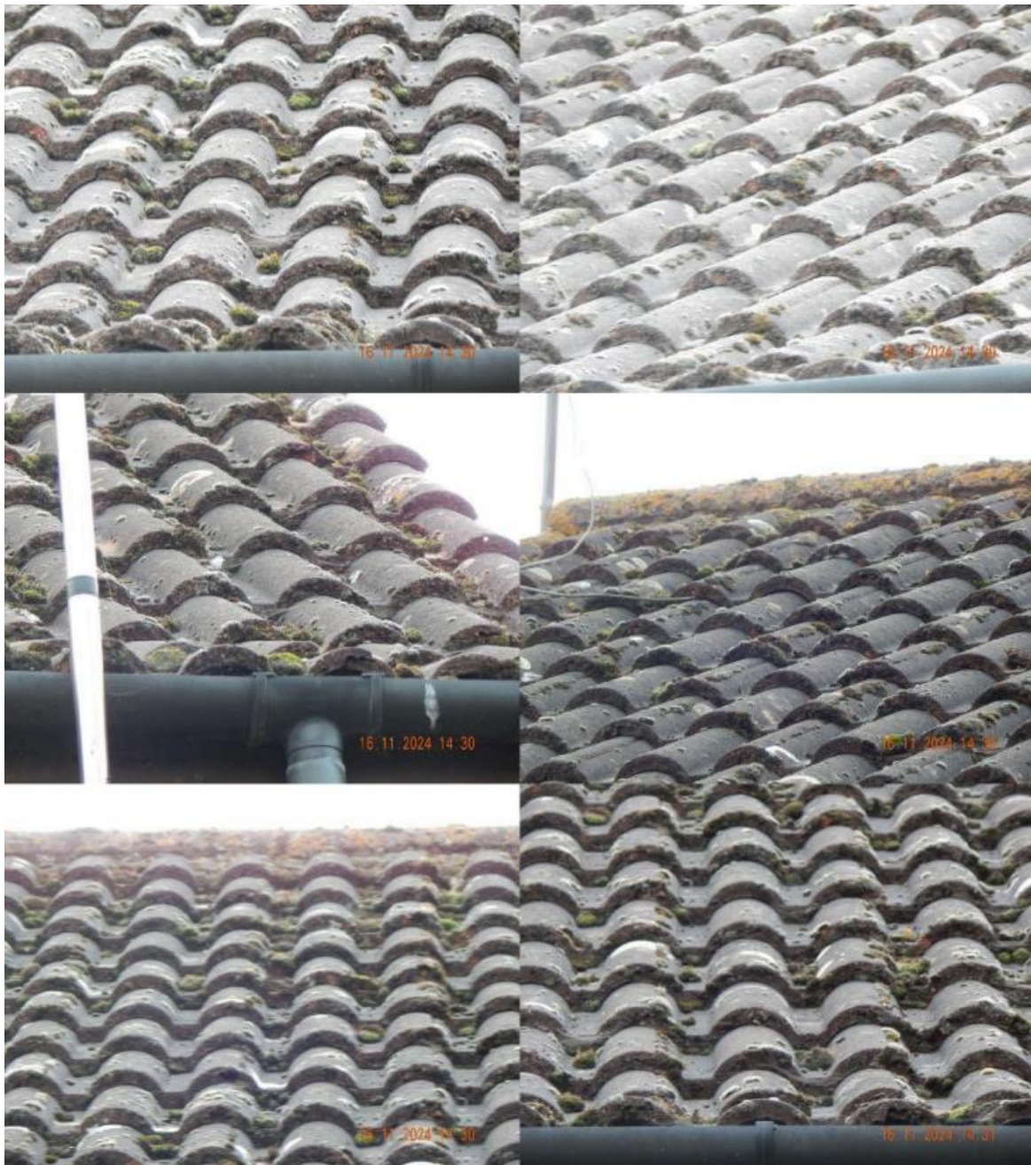
Image 5 – Close views of the upper and lower East facing roof coverings
