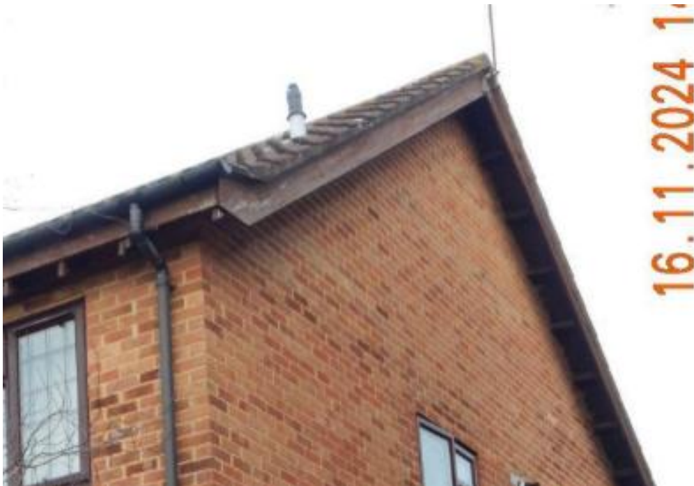
Image 7 – South facing elevation of the property
