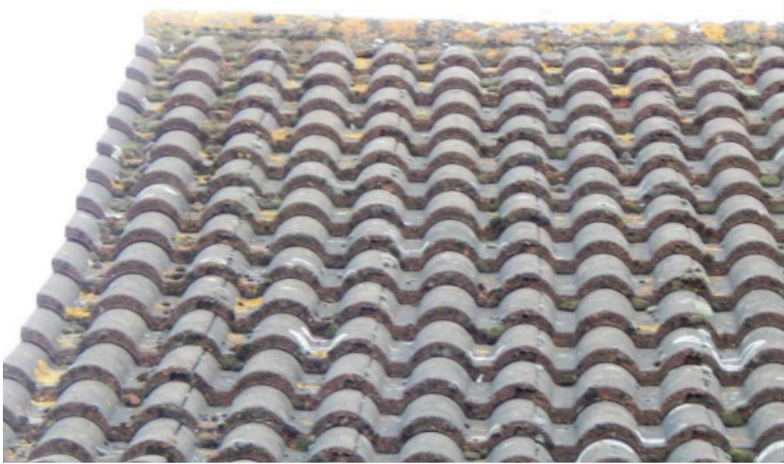
Image 3 – Close view of the upper West facing roof coverings to the property
