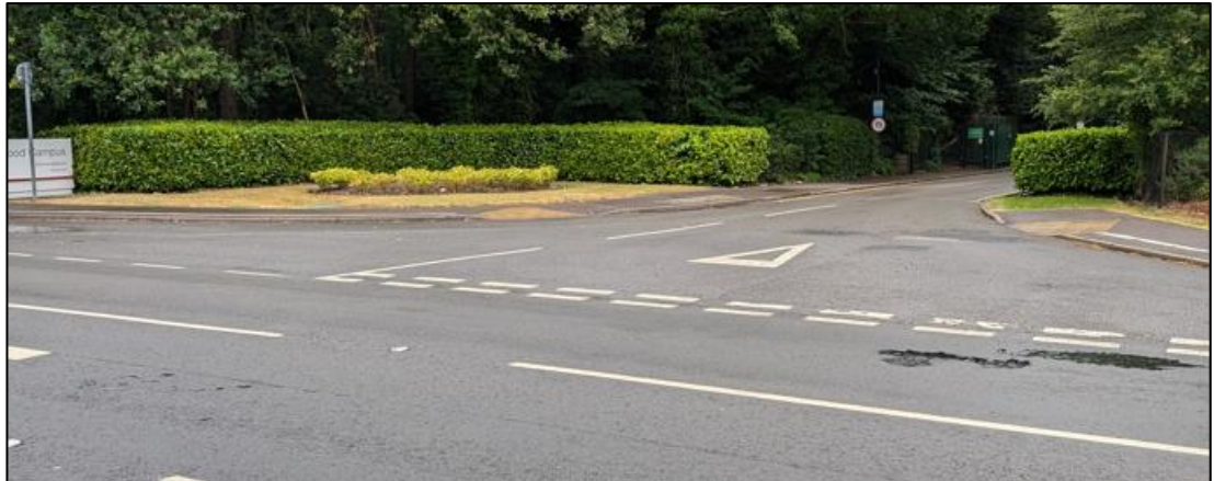
Image 3.2: Site Access / Nine Mile Ride Junction
