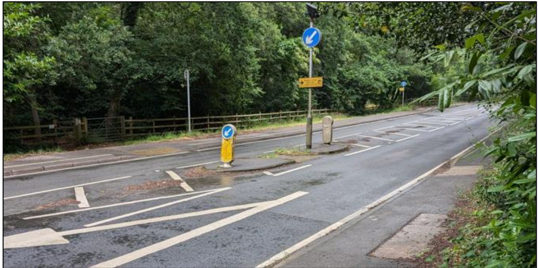
Image 3.1: Crossing Facility on Nine Mile Ride
