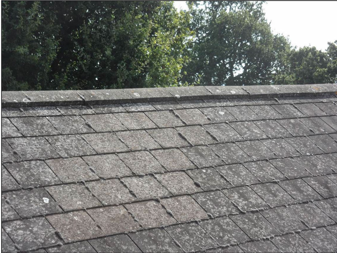
Figure 5. Example of ridge tiles. 8 Hunters Way, Spencers Wood, 28.08.24
