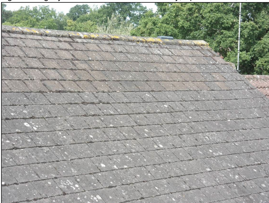
Figure 4. Tightly fitted roof tiles. 8 Hunters Way, Spencers Wood, 28.08.24
