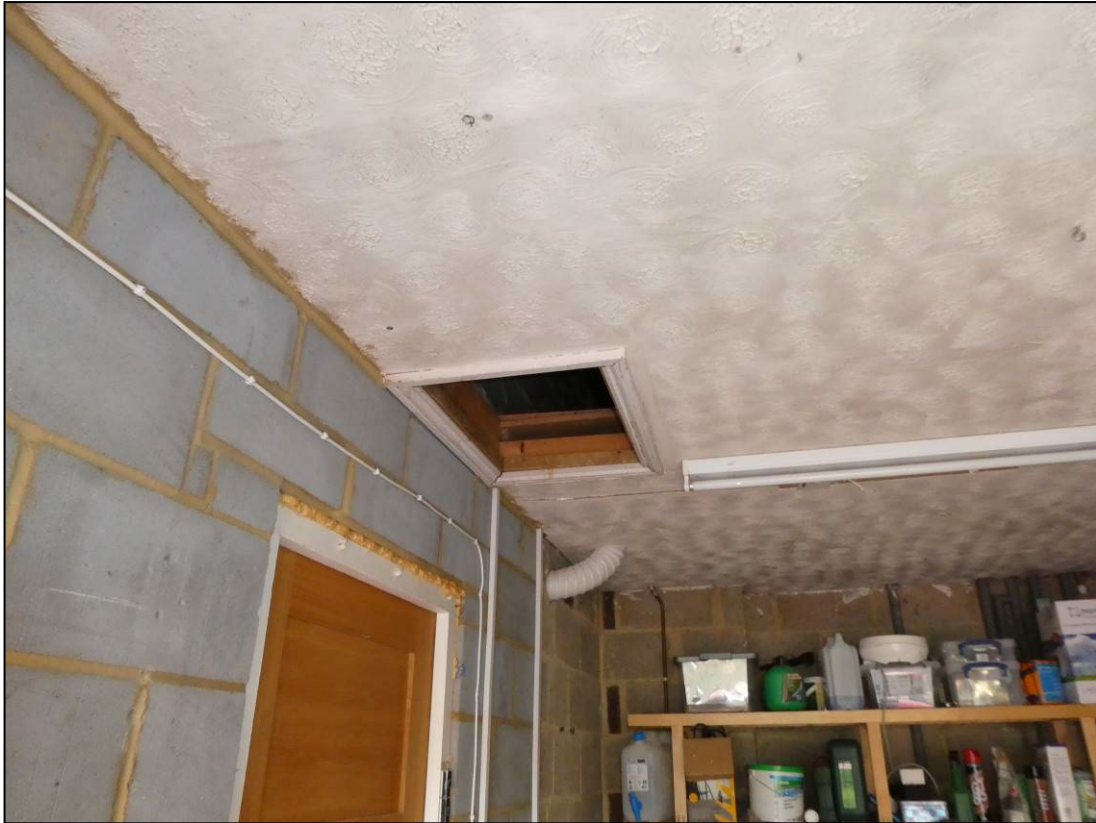
Figure 14. Example of loft hatch to garage loft. 8 Hunters Way, Spencers Wood, 28.08.24
