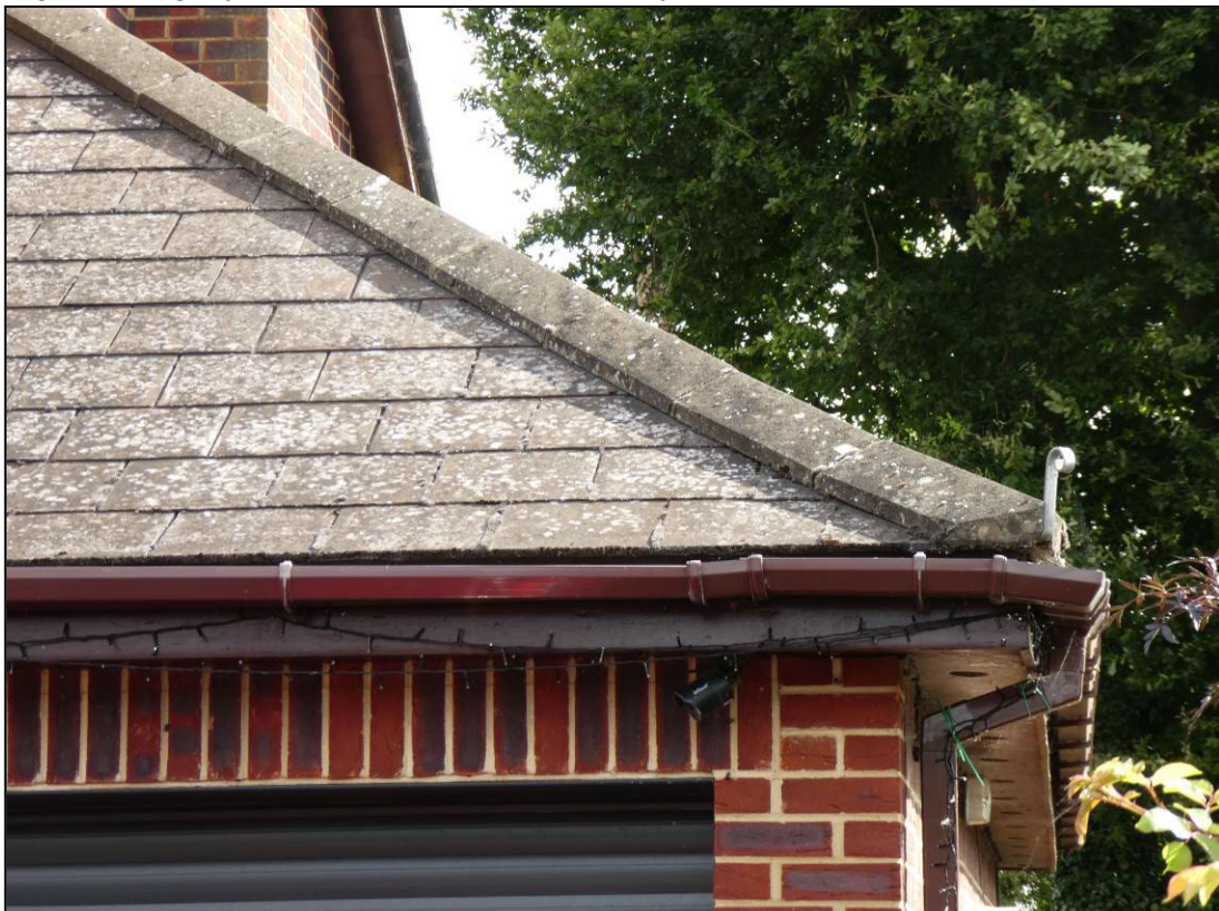
Figure 6. Tightly fitted hip tiles. 8 Hunters Way, Spencers Wood, 28.08.24
