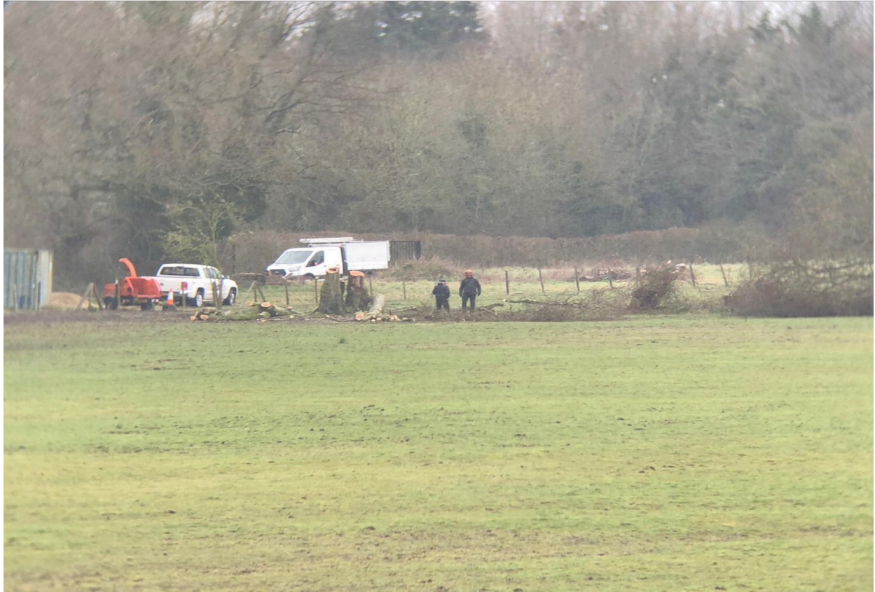
Image taken on 10-Mar-21 of the felling of two trees which would have stood in the way of the access road.
