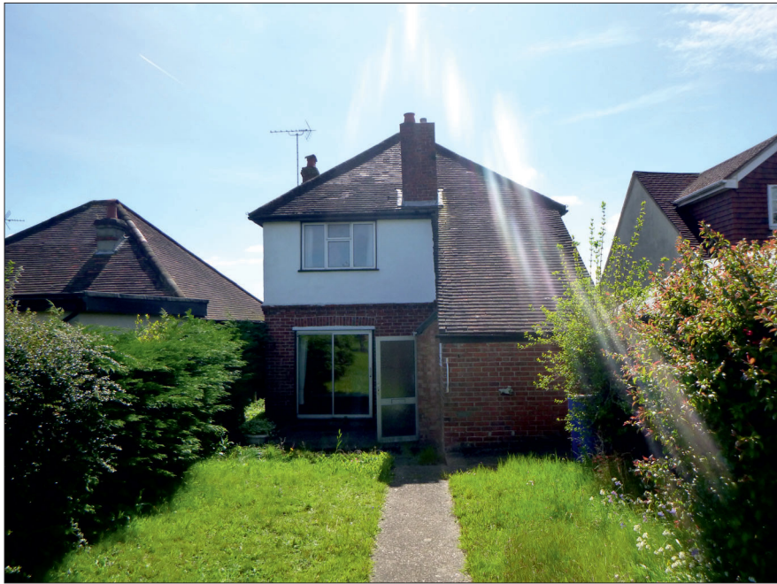
Photograph 2: Showing the rear of the building.
