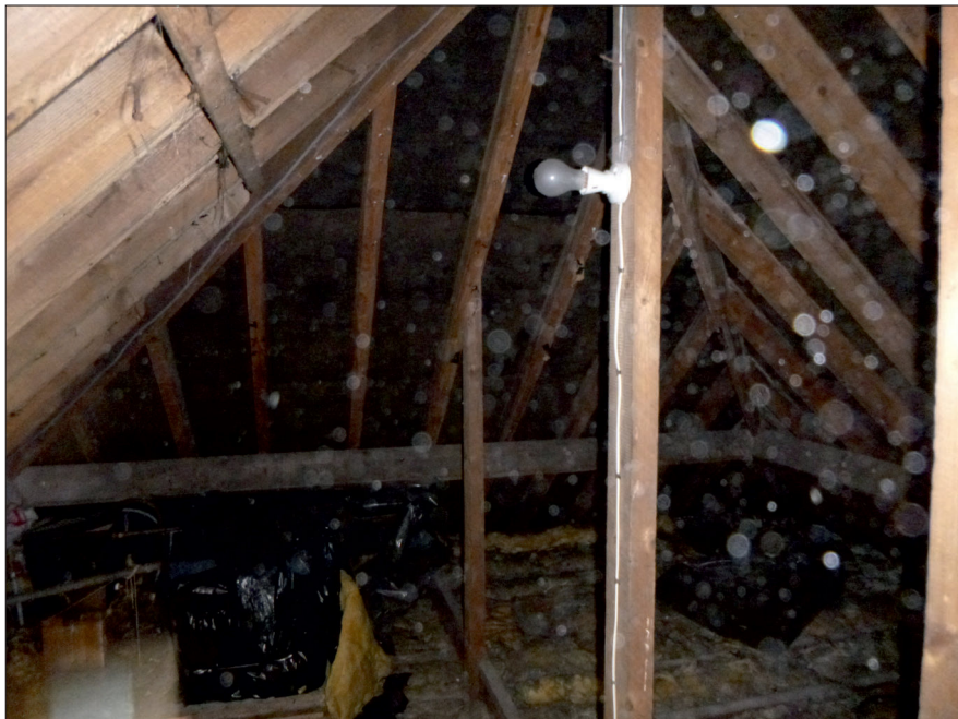
Photograph 3: Showing the single roof space, which was dusty and cobwebbed throughout.
