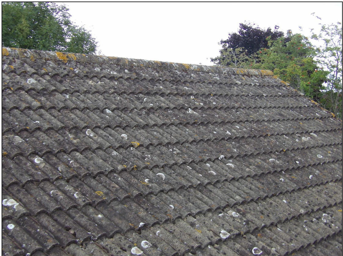
Figure 4. Tightly fitted roof and ridge tiles. 14 Eastbury Park, Winnersh. 22.07.25
