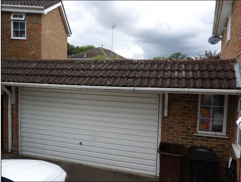
Figure 8. Tightly fitted roof and ridge tiles on false pitched roof of garage. 14 Eastbury Park, Winnersh. 22.07.25
