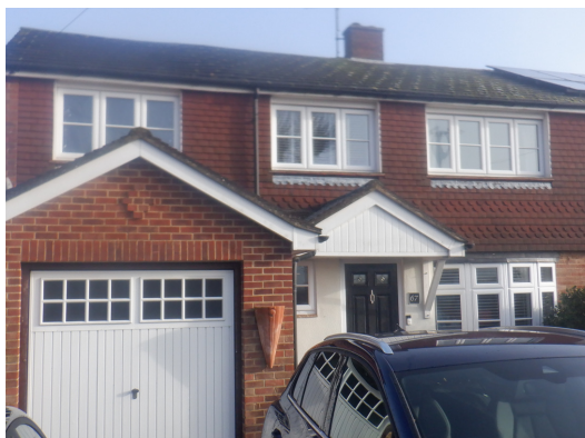
Photograph 10. Hanging tiles on front elevation.
