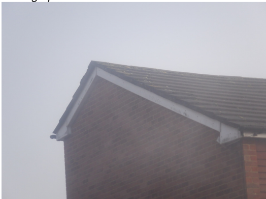
Photograph 7. Gable verge mortar intact.
