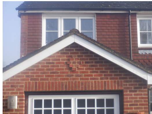
Photograph 6. Garage gable verge mortar intact.
