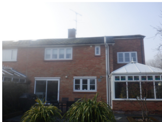
Photograph 2. Rear of property viewed from the northeast.
