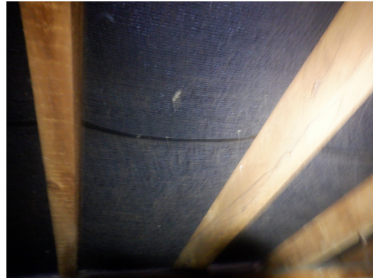
Photograph 18. Intact bitumen liner in newer extension section (TN8).
