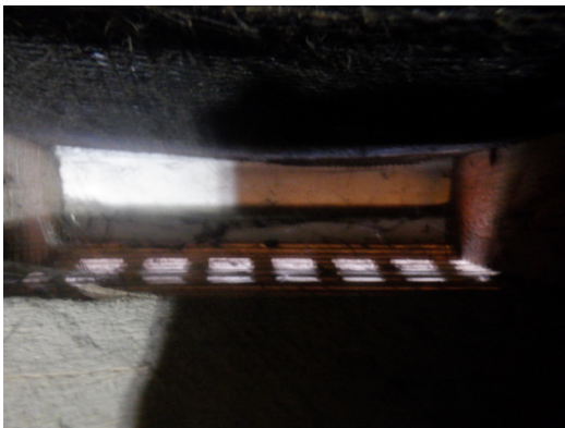
Photograph 21. Eaves open and vented soffits visible (TN13).
