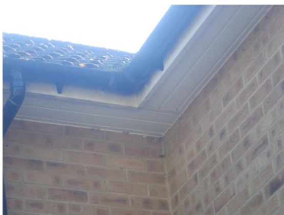
Photograph 12. uPVC soffit sealed to the brickwork walls of the building.
