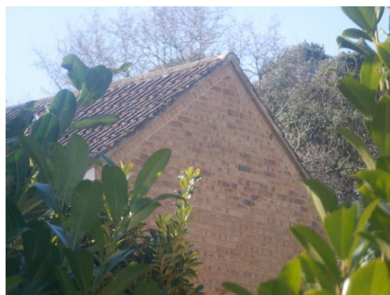
Photograph 4. Intact verge mortar along the gable (east elevation).
