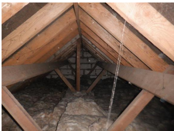
Photograph 13. Void of cut & pitch construction
