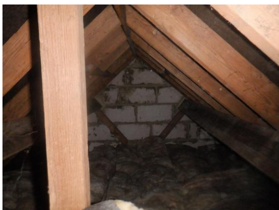
Photograph 16. northeastern blockwork gable fully sealed to the timbers.
