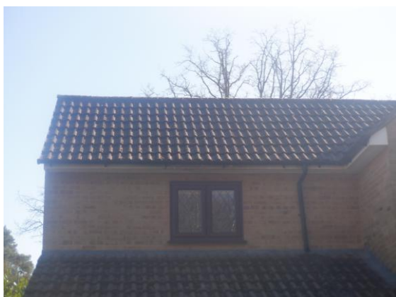
Photograph 3. Fully sealed interlocking roof tiles (rear elevation).
