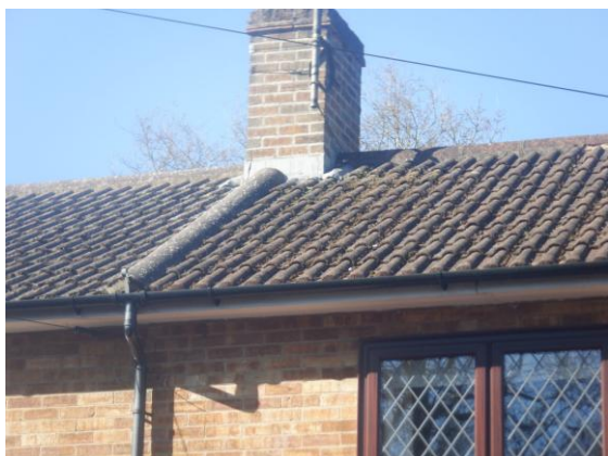
Photograph 9. Lead flashing sealed at the base of the chimney (front elevation).
