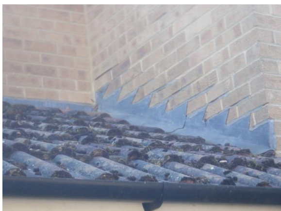
Photograph 11. Lead flashing sealed to the brickwork wall and roof tiles (rear elevation).
