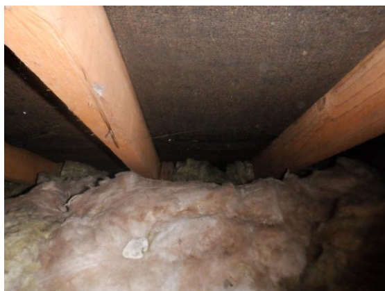
Photograph 15. Eaves filled with fibreglass insulation.
