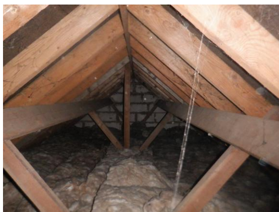
Photograph 17. Northern blockwork gable fully sealed to the timbers.
