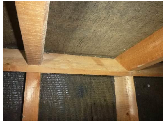
Photograph 10. Bitumen roof lining.
