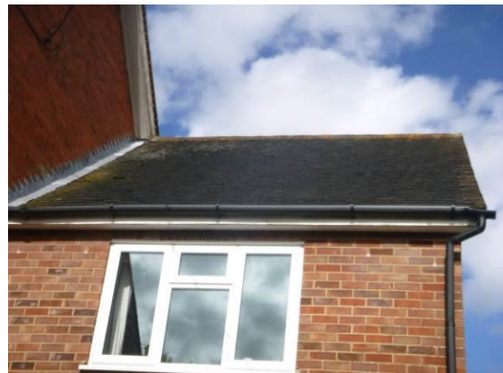
Photograph 3. Overlapping plain tiles on extension (front elevation).
