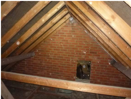
Photograph 9. Side extension roof void.
