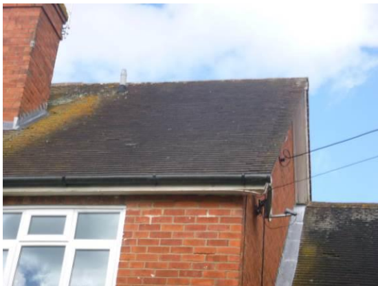
Photograph 2. Overlapping plain tiles (front elevation).
