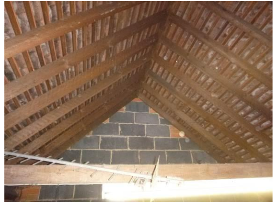
Photograph 8. Unlined roof.
