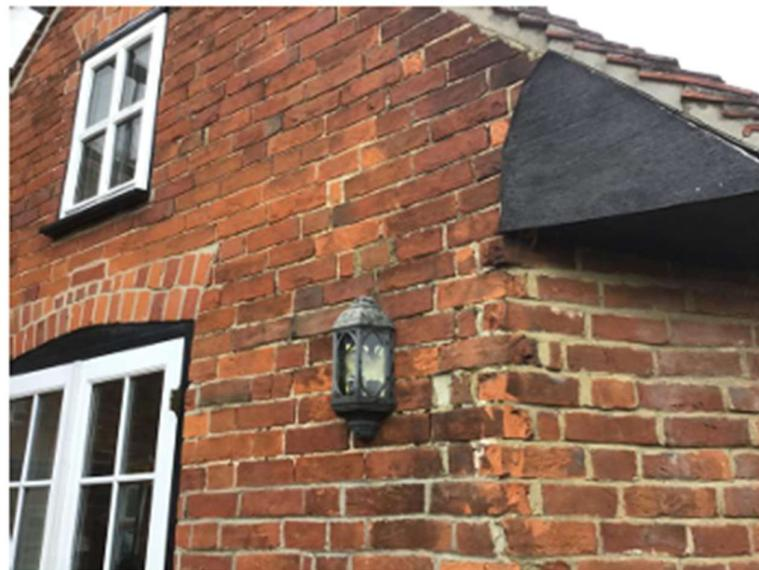
The North elevation has been poorly pointed in a hard sand and cement mortar, raised beyond the brick face. This inappropriate material has compromised the breathability of the historic fabric. It is therefore proposed that the cementitious pointing be carefully removed and replaced with lime mortar, in the same manner as outlined above, to restore the building's natural performance and ensure long-term preservation.
