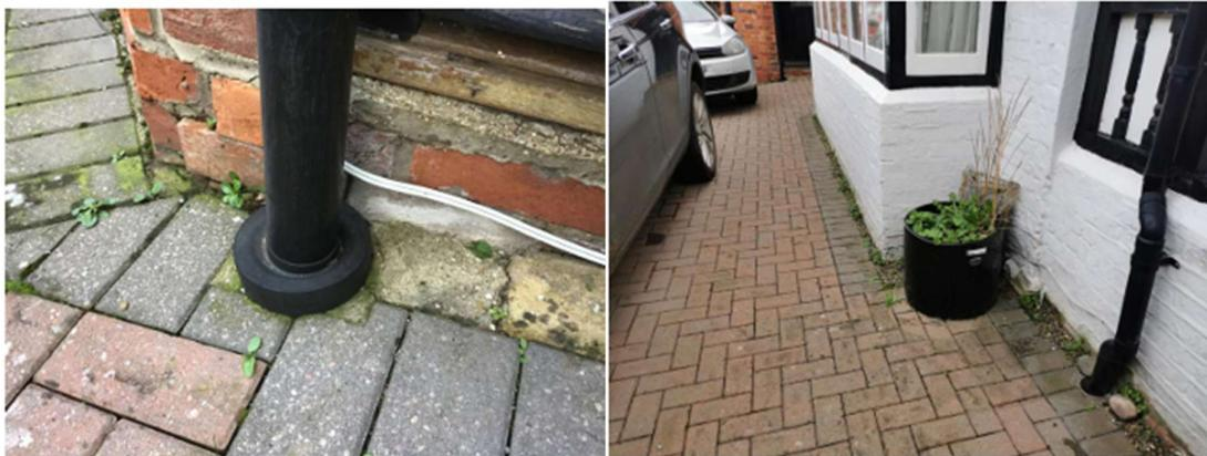
To address damp issues, it is proposed the paving be cut back to a minimum 100mm from the walls and replaced with a shingle French drain or slot drain connected to the surface water system. This measure will improve breathability, protect the building fabric, and safeguard the long-term integrity of the heritage asset against damp.
