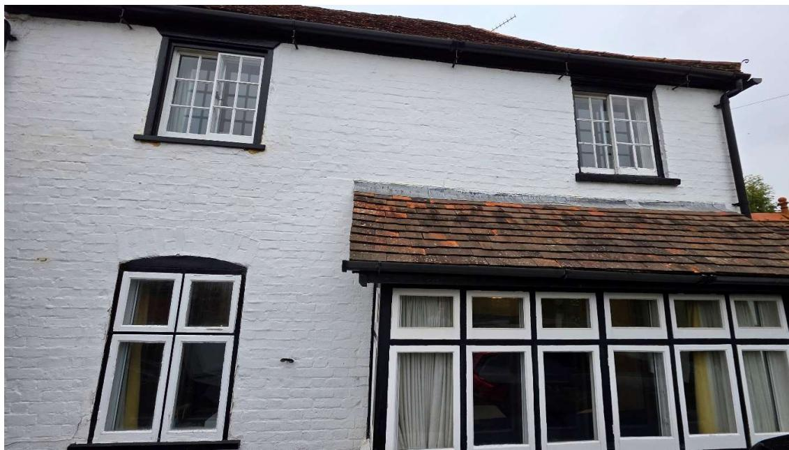
To support the application, a Method Statement and Recommendation for the use of the Stonehealth Steam DOFF system has been included. This recognised conservation technique for masonry and building fabric provides a controlled approach to the removal of soiling and non-breathable coatings, ensuring the brickwork is cleaned without damage and the historic fabric is protected.
