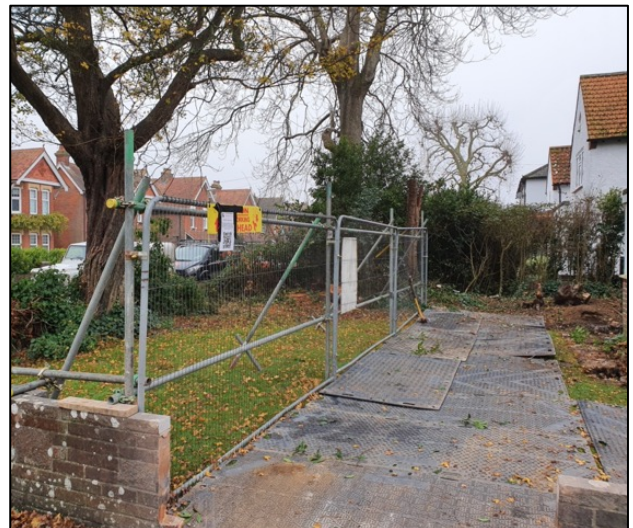
GP2: Tree protection barriers & trackmat ground protection
