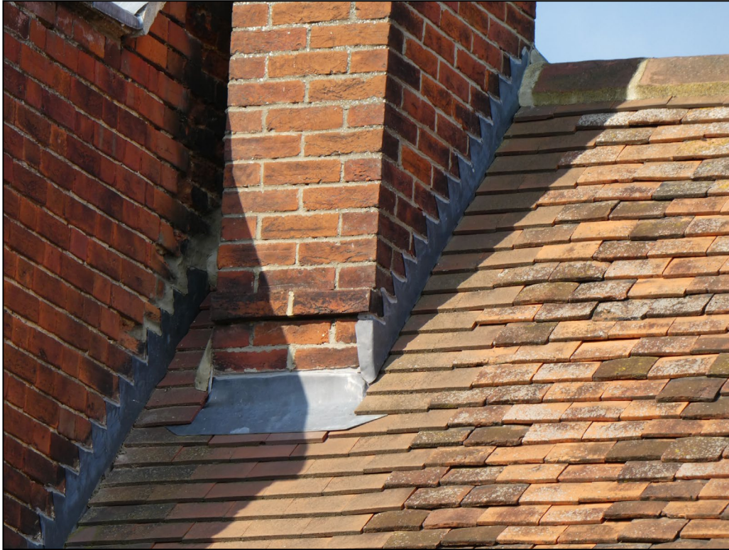
Figure 9. Example of sealed lead flashing. 36/38 Rose Street, Wokingham. RG40 1XU
