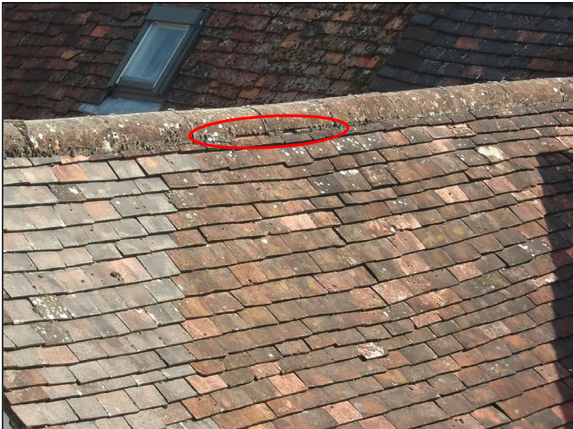
Figure 6. Example missing mortar from ridge tiles. 36/38 Rose Street, Wokingham. RG40 1XU
