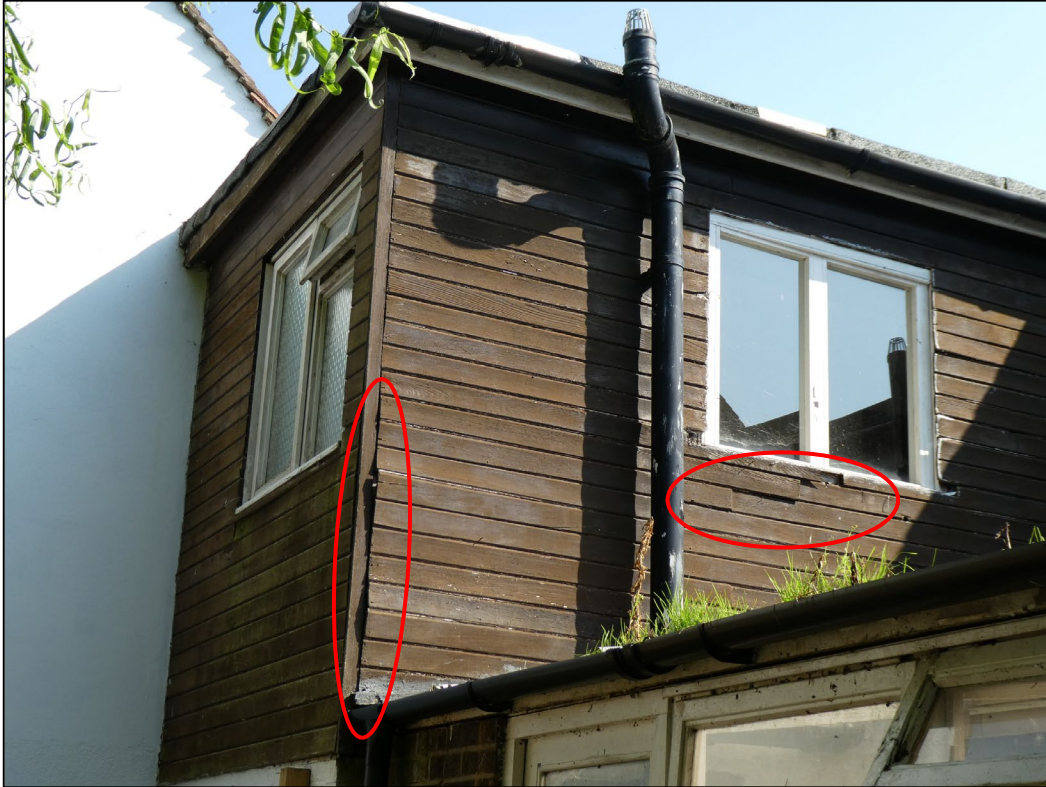
Figure 11. Rear, timber clad 1 st floor extension with warped cladding. 36/38 Rose Street, Wokingham. RG40 1XU
