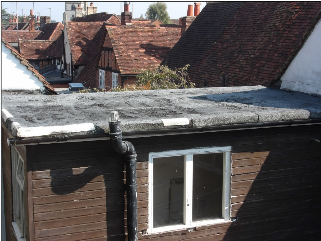
Figure 12. Roof of timber clad extension. 36/38 Rose Street, Wokingham. RG40 1XU
