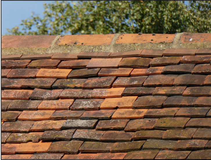
Figure 5. Example raised/lifted roof tiles. 36/38 Rose Street, Wokingham. RG40 1XU
