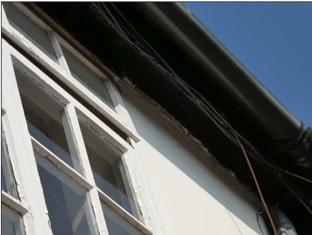
Figure 10. Example sealed soffits and fascias. 36/38 Rose Street, Wokingham. RG40 1XU
