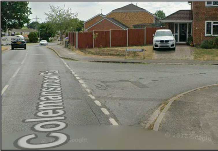
Photo 2: View towards adjacent junction at Crediton Close showing a boundary fence positioned adjacent to the highway
