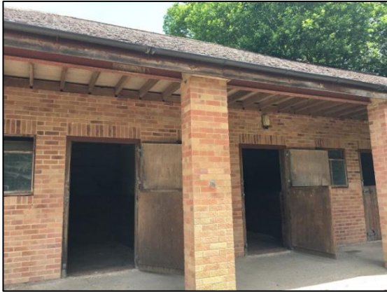
Photo 45 Barn structure (B3)
