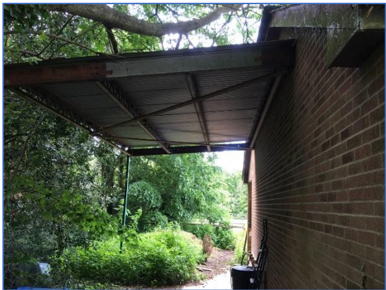
Photo 47 Barn structure (B3)
