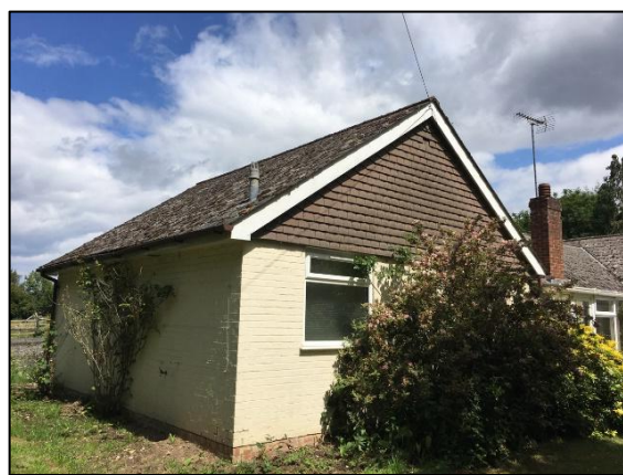
Photo 36 Residential dwelling (B1)
