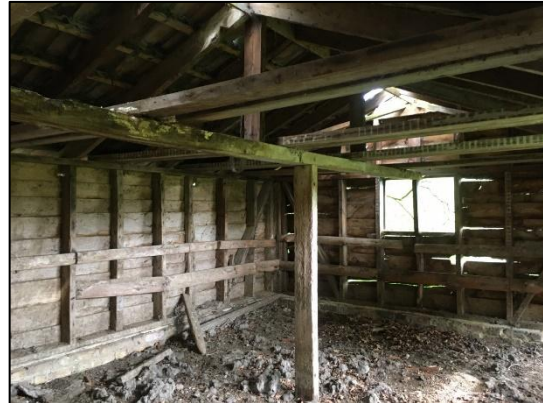
Photo 64 Timber outbuilding internals (B7)
