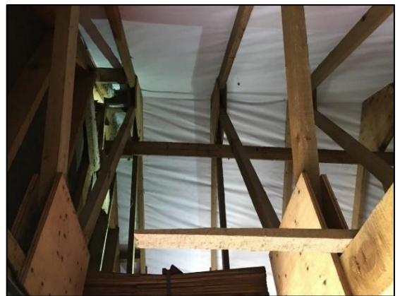
Photo 44 Internals of outbuilding (B2)
