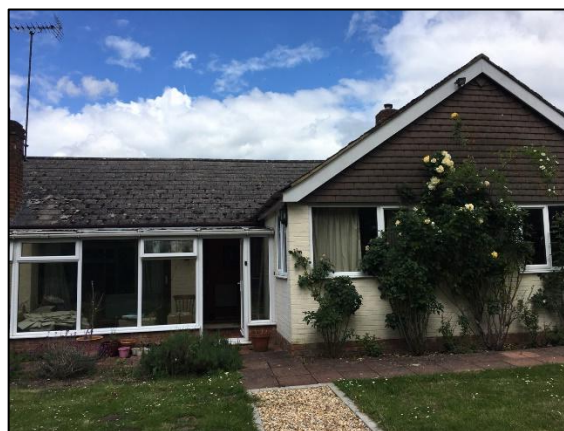
Photo 34 Residential dwelling (B1)
