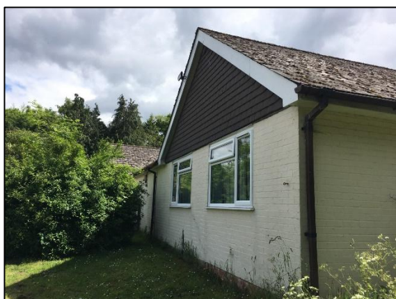
Photo 35 Residential dwelling (B1)
