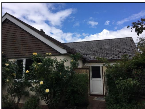
Photo 33 Residential dwelling (B1)
