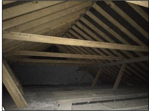
Photo 52 Barn loft void (B3)
