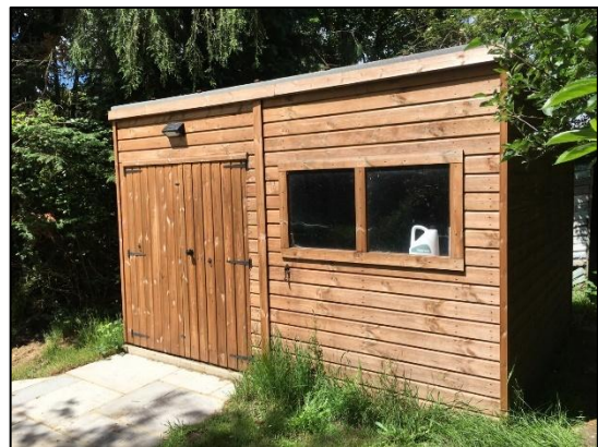
Photo 60 Timber shed (B6)
