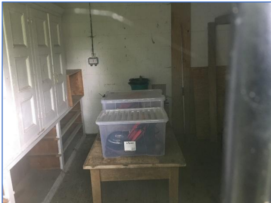
Photo 49 Storage room (B3)
