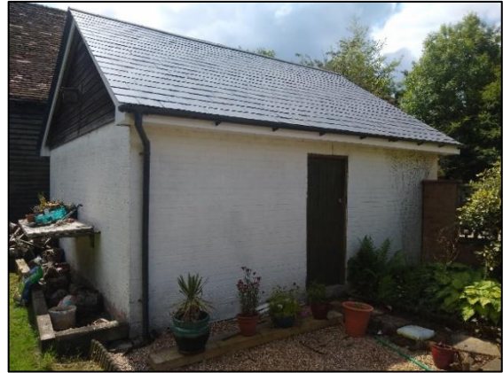
Photo 40 Brick outbuilding (B2)
