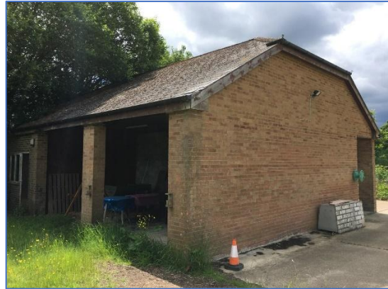
Photo 46 Barn structure (B3)
