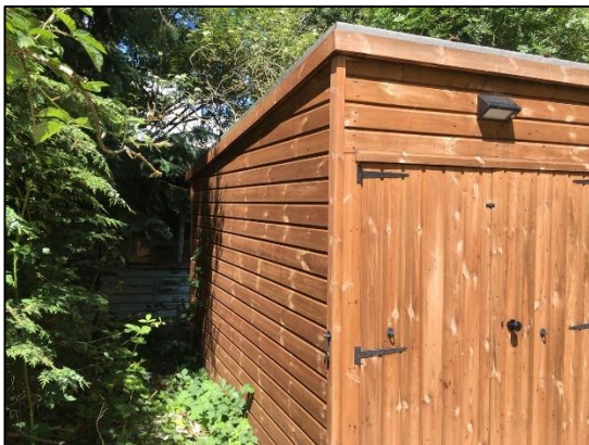
Photo 61 Timber shed (B6)
