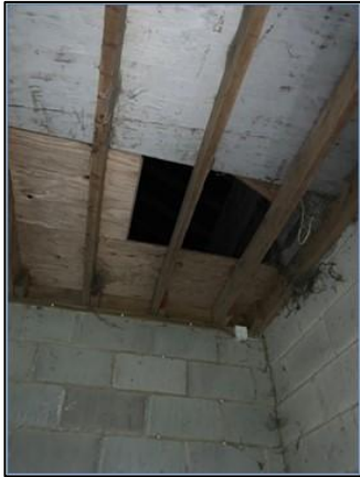
Photo 51 Loft hatch used as an entrance by BLE bats
