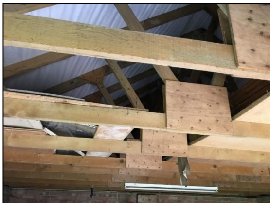
Photo 43 Internals of outbuilding (B2)
