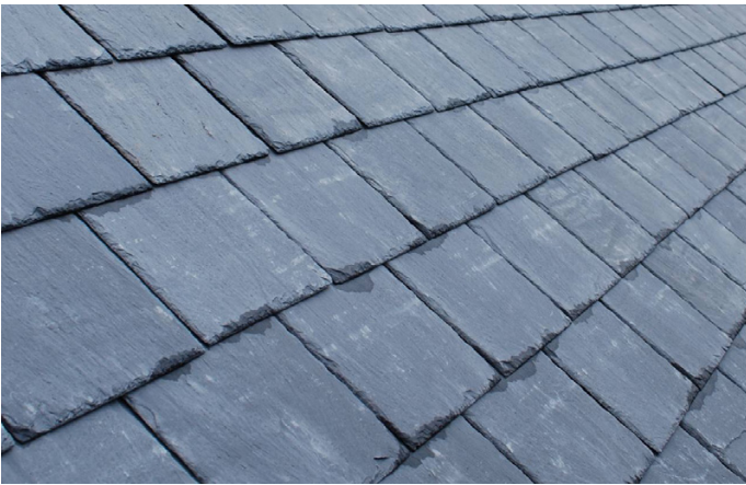
Roof - Natural Slate
