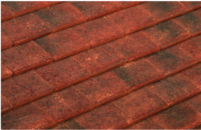
Roof - Red Clay Tile
