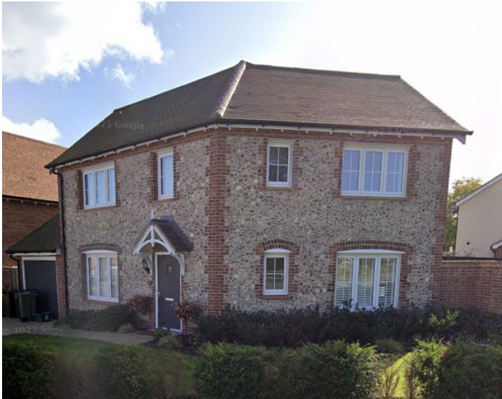
Materiality of random knapped flint as included on some plots at Bridge Farm, Twyford
