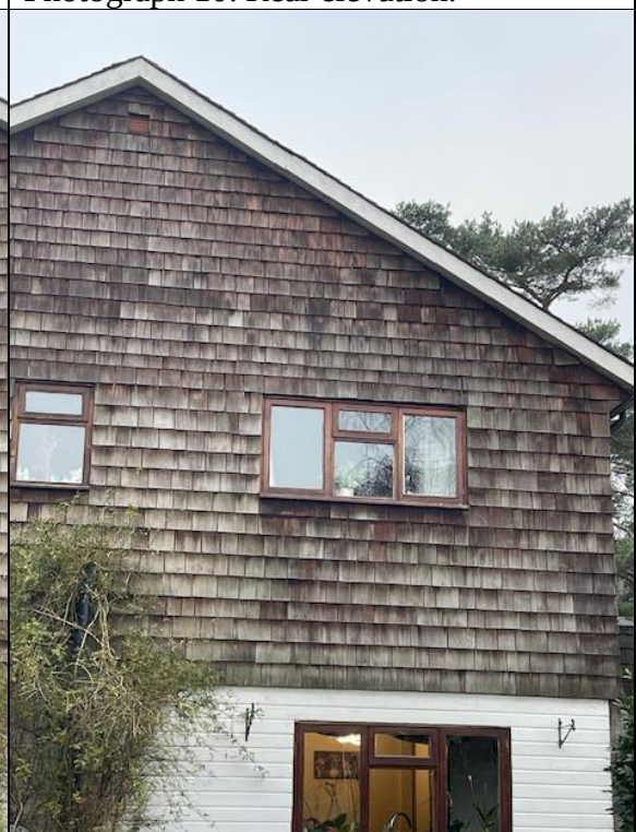
Photograph 12: Cedar cladding around the building.
