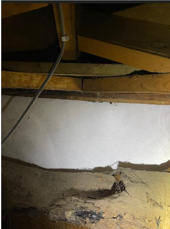
Photograph 5: Hanging tiles. Loft space.
