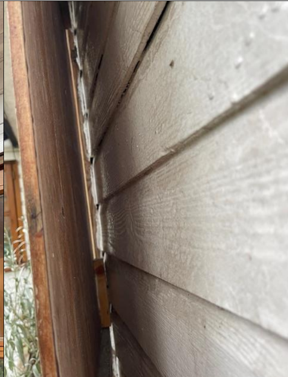
Photograph 22: No gaps around cladding.
