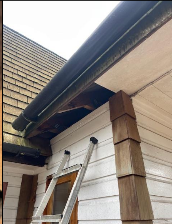
Photograph 14: Gaps around porch could be checked using a ladder, torch and endoscope.
