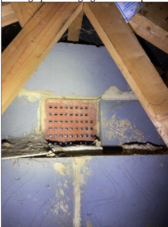
Photograph 7: Loft space-ventilation brick.
