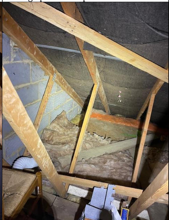
Photograph 8: Fibreglass insulation.
