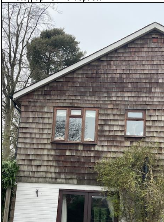
Photograph 11: Cladding tight and flat.
