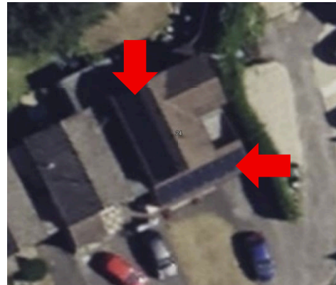
Bing aerial photograph of the roof configuration
