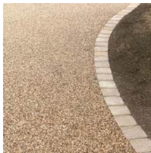
Setts edging to resin bound gravel
