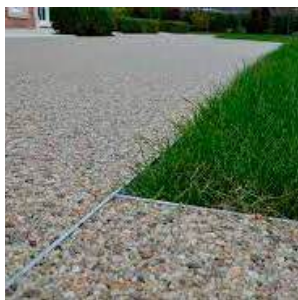
Aluminium edging to resin bound gravel
