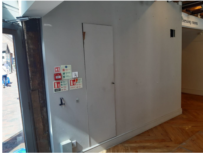
Stud wall covering fireplace (July 2020)
