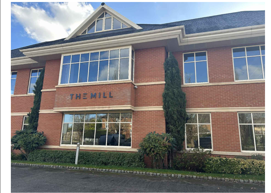
05 EXISTING EXTERIOR FRONT ELEVATION Photograph
