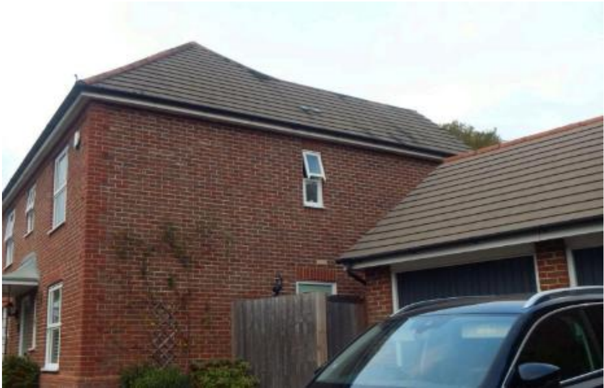
Image 3 – East facing elevation of the property
