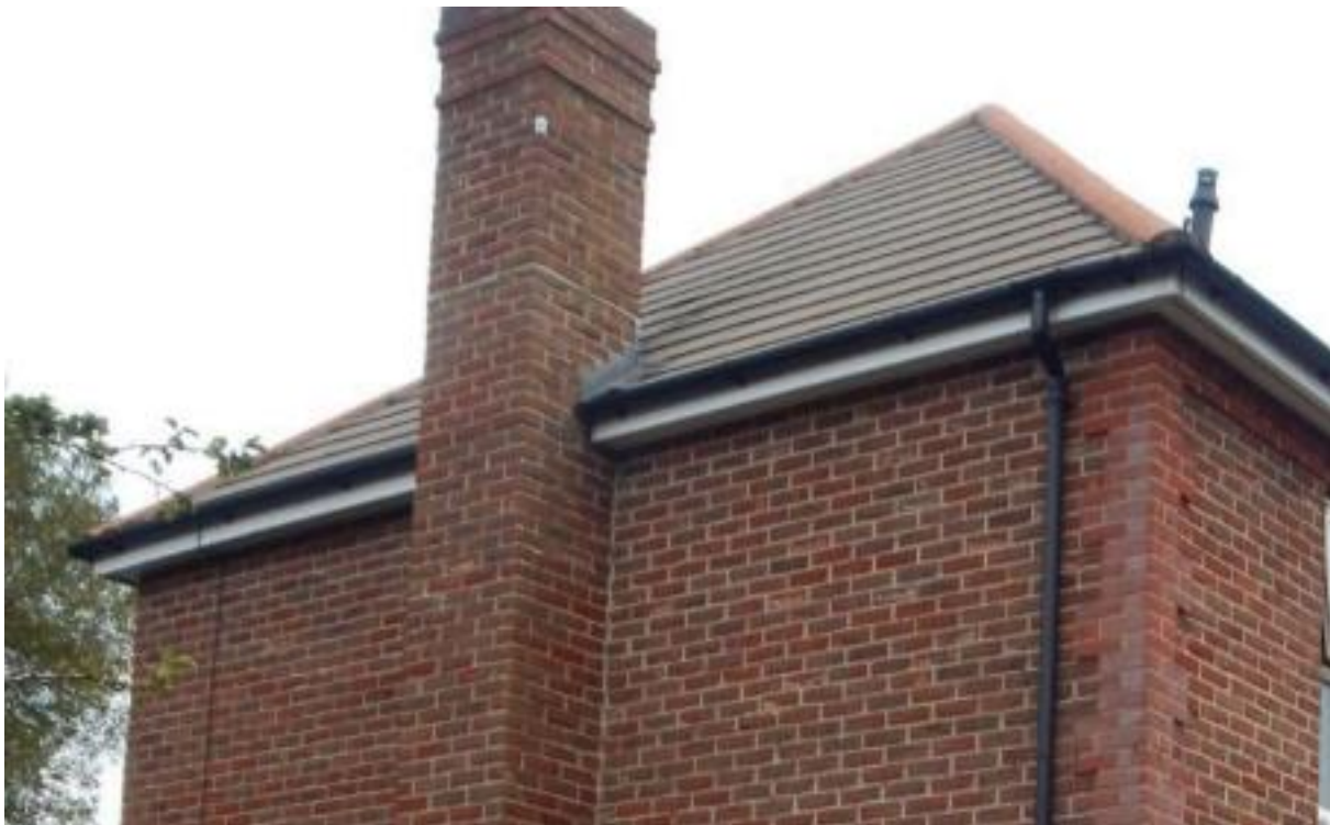
Image 4 – West facing elevation of the property
