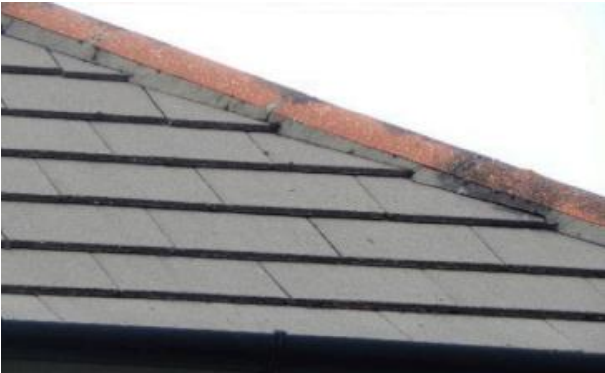
Image 6 – Close view of the main upper roof coverings to demonstrate condition throughout
