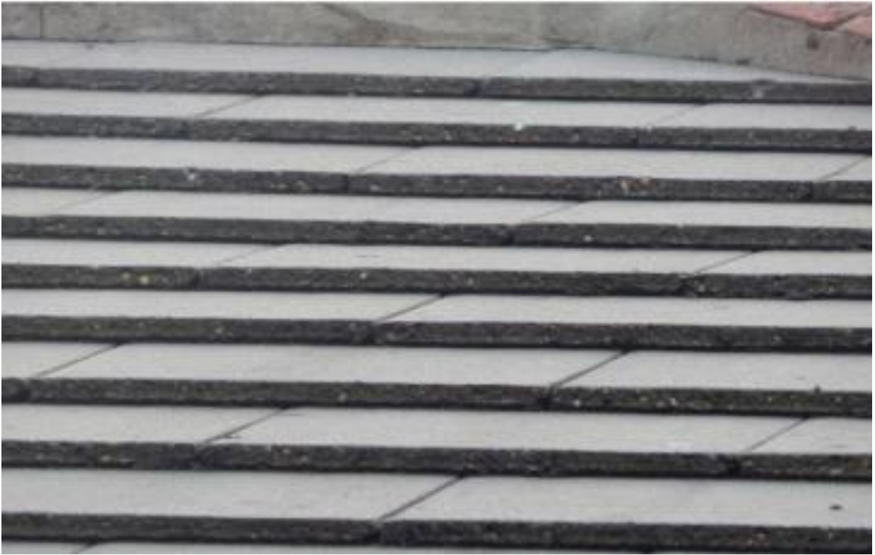
Image 5 – Close view of the main upper roof coverings to demonstrate condition throughout
