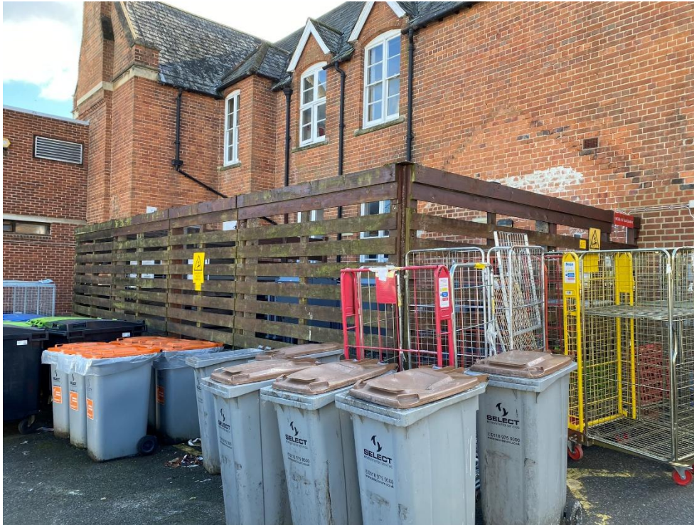
Photo 1 – View of existing Park House substation enclosure.
