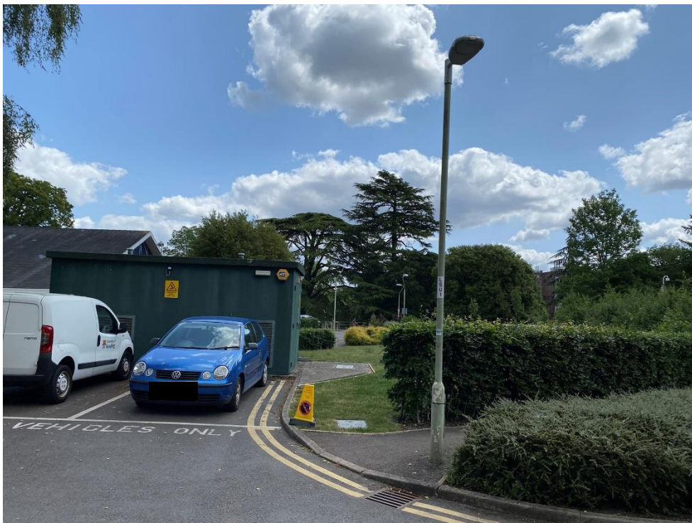
Photo 2 – View of existing Library substation building.
