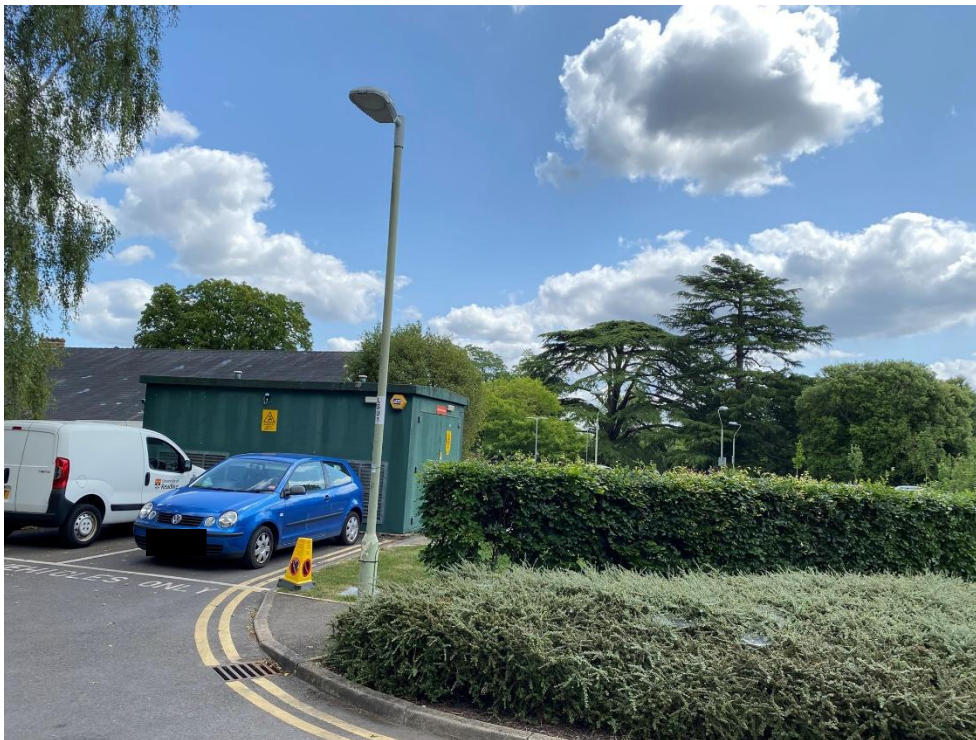
Photo 1 – Front elevation of existing substation
