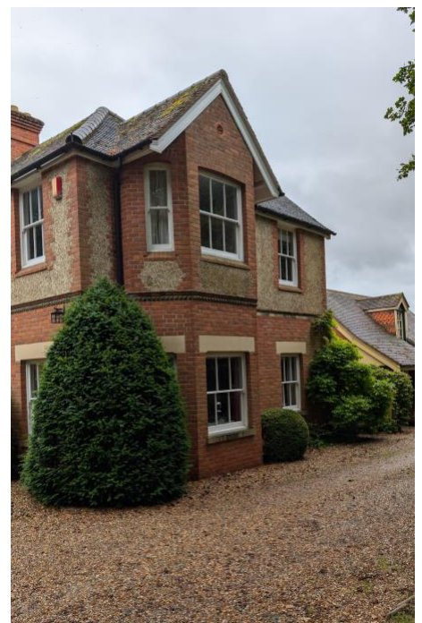
View of the West elevation (side), with the Coach House in the background
