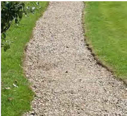
SELF-BINDING GRAVEL FOOTPATH
