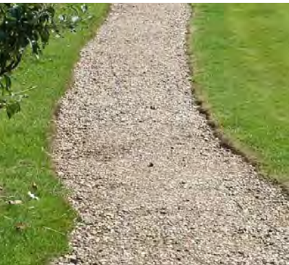
SELF-BINDING GRAVEL FOOTPATH
