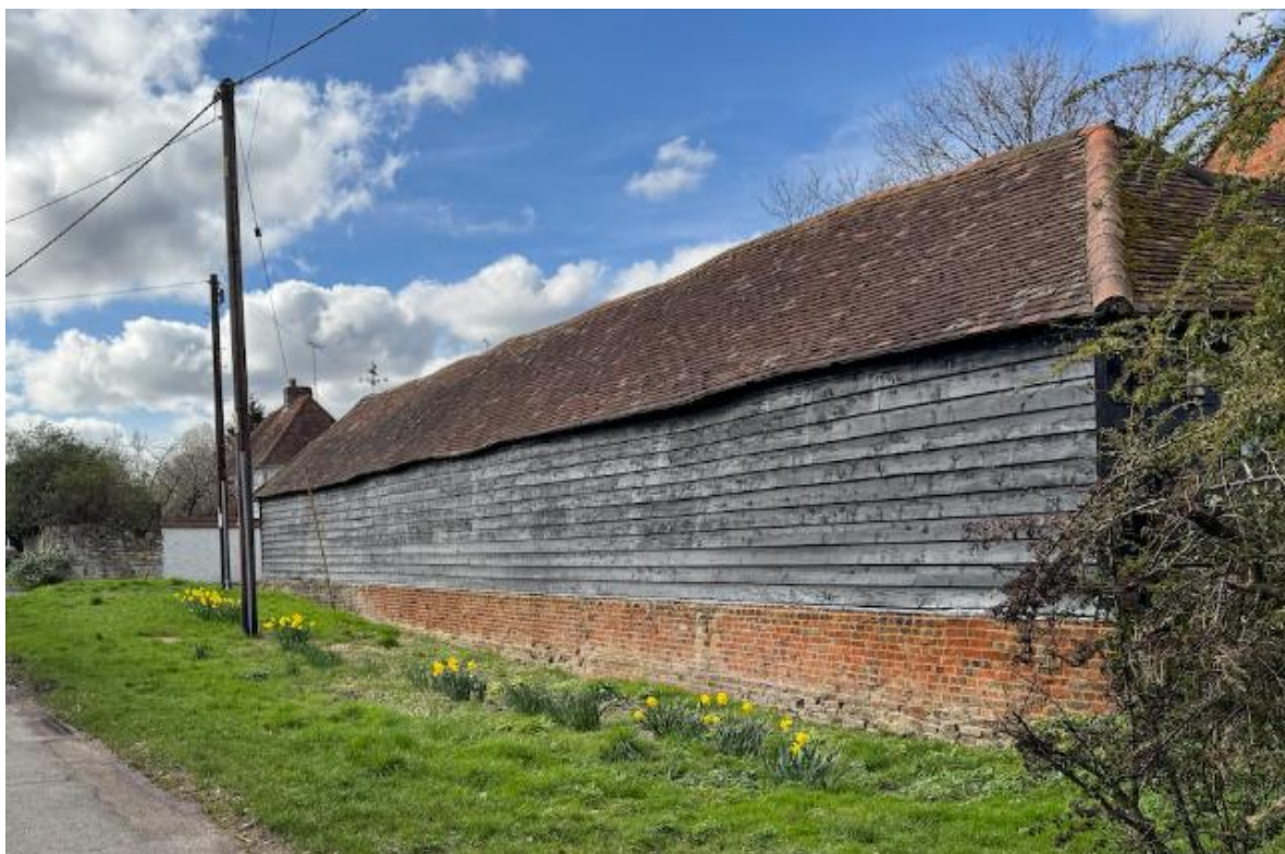
Fig. 11: View, looking west from Hogmoor Lane, of the road frontage of Long Barn.
