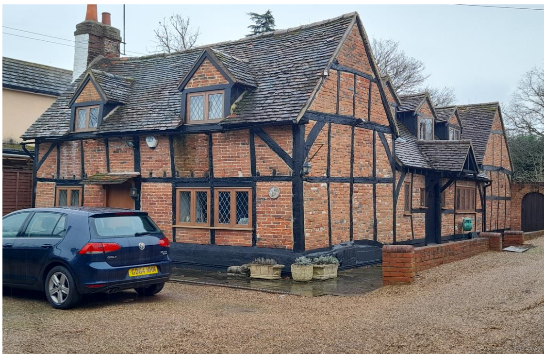
Fig. 5: View, looking south-east from Broadwater Lane, of Bower Cottage.
