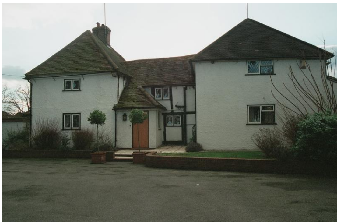
Fig. 8: View, looking south, of the rear elevation of Wards Cross House (Historic England).
