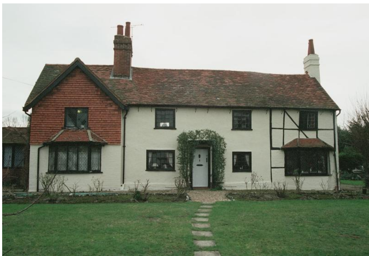
Fig. 4: View, looking south-west, of the main front of Buttercups (Historic England).
