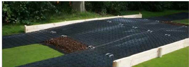
Fig. 3 Temporary Ground Protection Example
