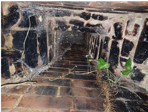
Plate 14: Chimney type structure on north elevation of northern wall
