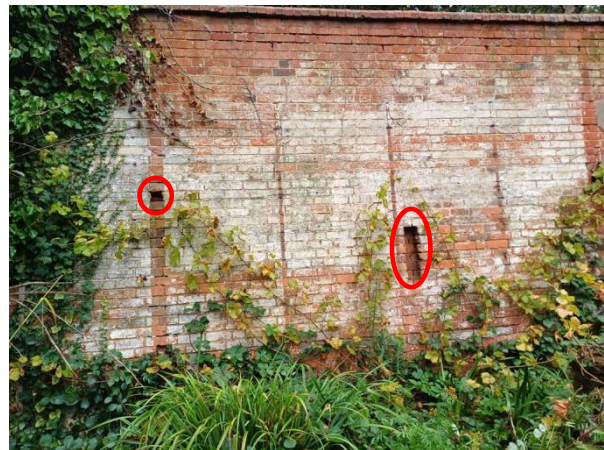
Plate 12: PRF's on interior southern elevation of northern wall (red circles)
