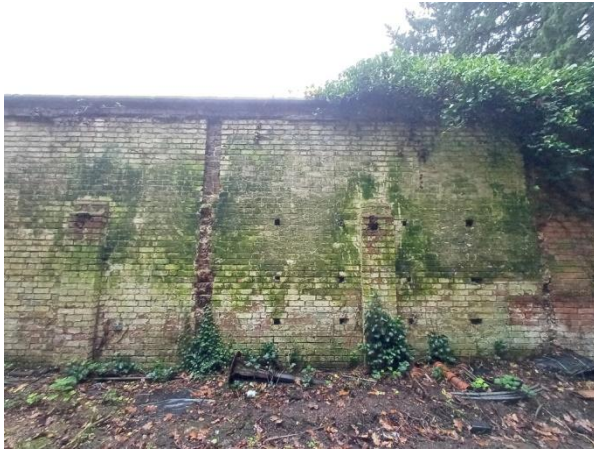
Plate 7: Gaps and potential bat roosting features and nesting bird habitat on exterior north elevation
