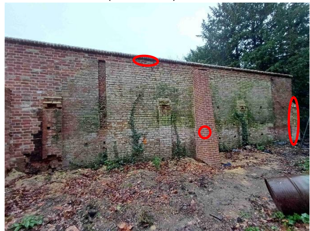
Plate 15: New butress blocking PRF, repointed coping bricks and removal of thick-stemmed ivy
