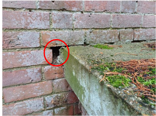
Plate 13: PRF on interior western elevation of eastern wall (red circle)
