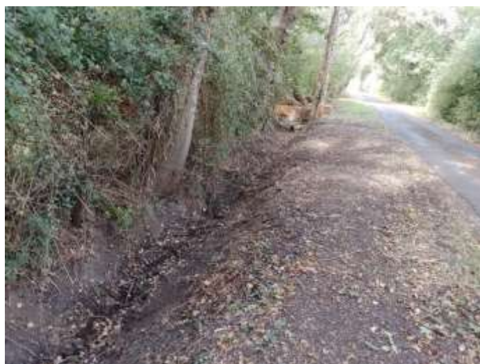
Figure 3: Access and drainage ditch along Nelson Lane
