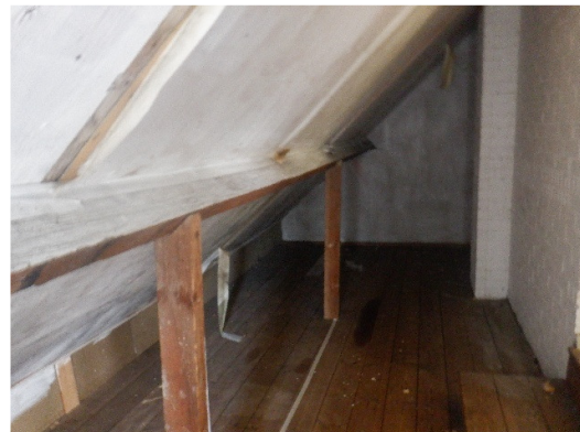
Photograph 22. Eaves space viewing west (Eave space).
