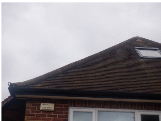
Photograph 3. Roof, hip and ridge tiles flat and sealed (rear elevation).
