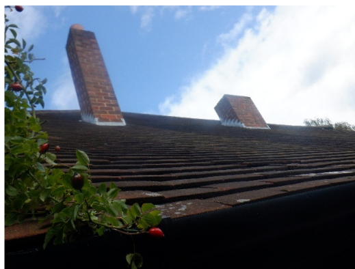
Photograph 4. Lead flashing tight around the chimneys (south elevation).
