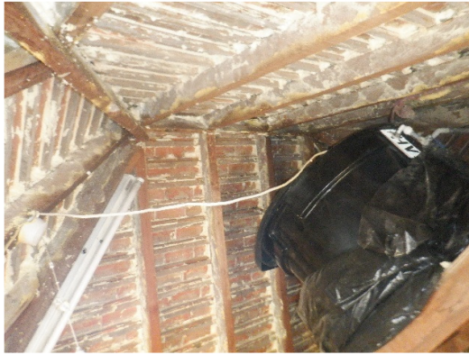
Photograph 16. Expanding foam between the tiles (First roof void).
