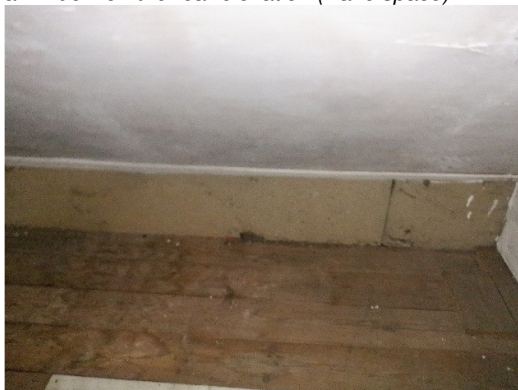
Photograph 23. Floor boarded with timber panels and eaves boarded (Eave space).
