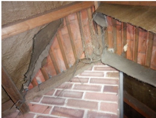
Photograph 18. Second roof void.
