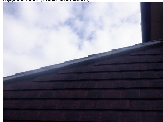
Photograph 10. Verge fully mortared on the single storey extension (front elevation).
