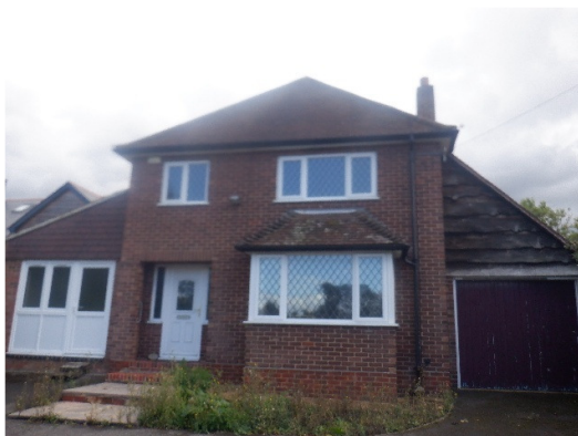
Photograph 1. Front of property viewed from east.
