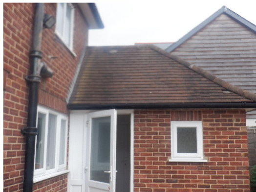
Photograph 7. Tightly fitted roof, ridge and hip tiles on the single storey side extension (rear elevation).
