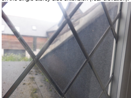
Photograph 9. Section of roof lined with bitumen felt (northern elevation).
