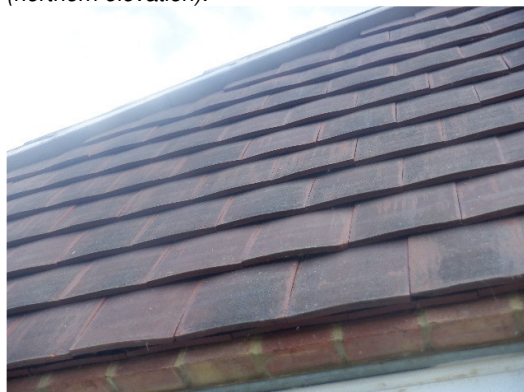
Photograph 11. Tight hanging tiles on the single storey extension (front elevation)
