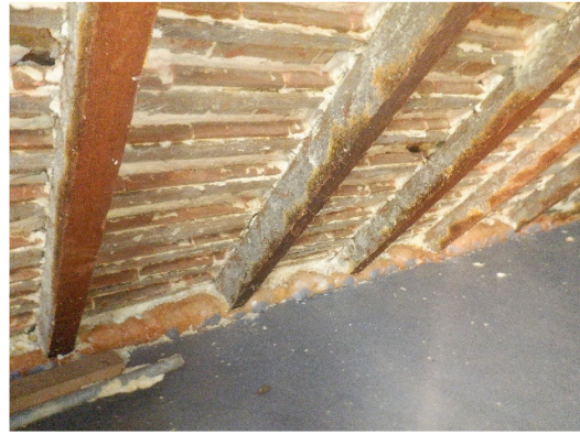
Photograph 17. Expanding foam filling the eaves (First roof void).
