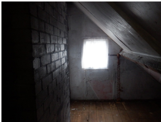
Photograph 21. Eave space above the garage with a window on the rear elevation (Eave space).
