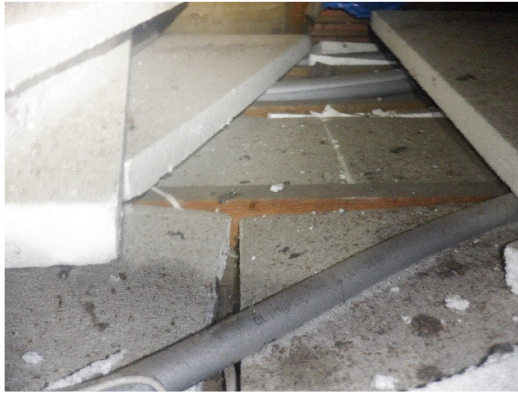
Photograph 20. Polystyrene blocks on the floor (Second roof void).
