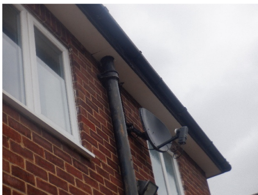
Photograph 5. Timber soffits tight to the brickwork (rear elevation).
