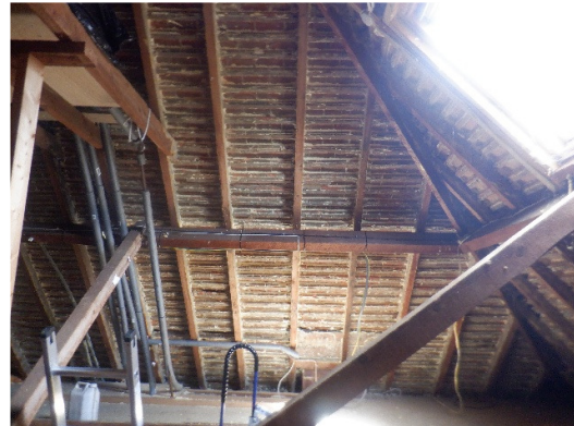
Photograph 15. Roof void illuminated with the roof light (First roof void).
