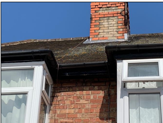
Photograph 5 (left). Well-sealed lead flashing around the chimney base. Photograph 6 (right). Fascia boards well sealed and hanging tiles that are not be impacted.
