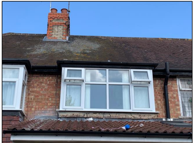
Photograph 3 (left). An example of a small gap the eaves. Photograph 4 (right). Clay roof tiles with a number of gaps that could potentially be used by crevice roosting bat species.
