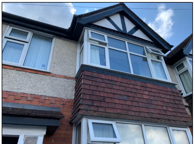
Photograph 5 (left). Well-sealed lead flashing around the chimney base. Photograph 6 (right). Fascia boards well sealed and hanging tiles that are not be impacted.
