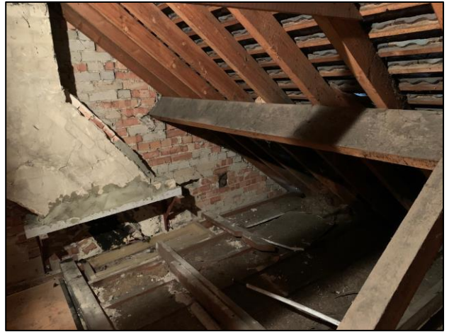
Photograph 1 and 2. The internal aspects of the void, showing the lack of bitumen lining and the rockwool insulation.
