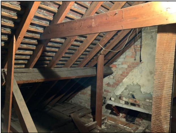
Photograph 1 and 2. The internal aspects of the void, showing the lack of bitumen lining and the rockwool insulation.
