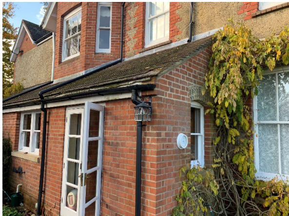
Pitched roof above existing kitchen.
