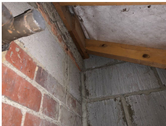
Roof membrane and well-sealed brick/block work.
