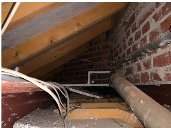
Roof space with exposed timbers and services.
