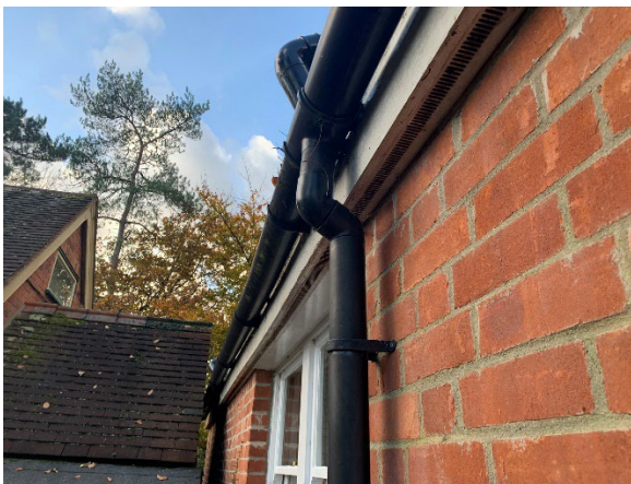
Well-sealed soffits to external brickwork.
