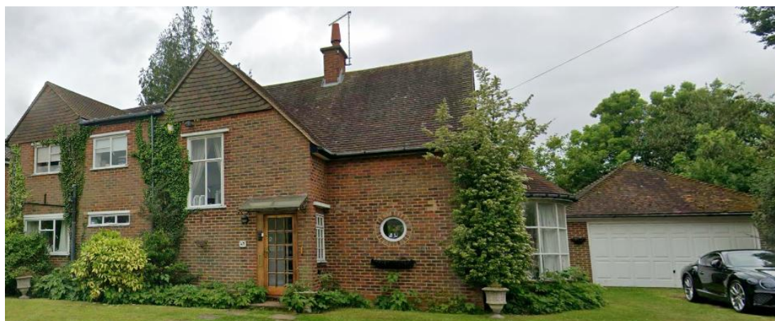
Front view of the current property
