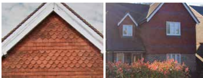
Decorative Tile hanging to highlight gables and key features
