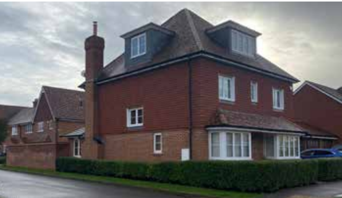
Detached house addressing the corner.
