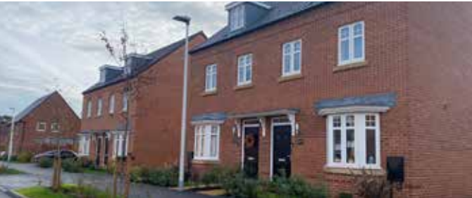
2.5 storey semi-detached houses.
