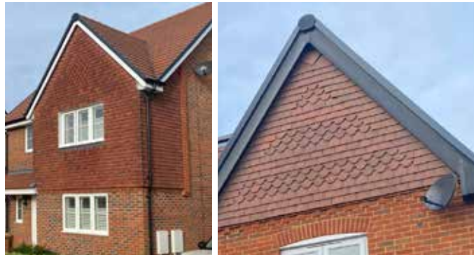
Tile hanging used to highlight key features.
