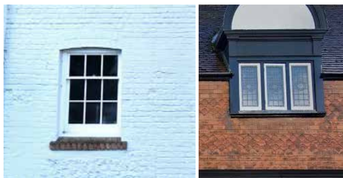
Light Painted brick
