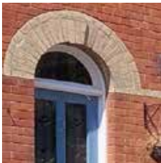
Contrasting brick for decorative details
