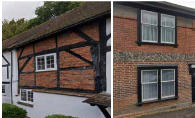
Timber frame with Brick infill
