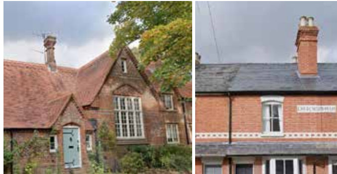
Clay and slate roof tile and red brick walls
