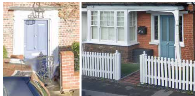
Panelled doors and bay window
