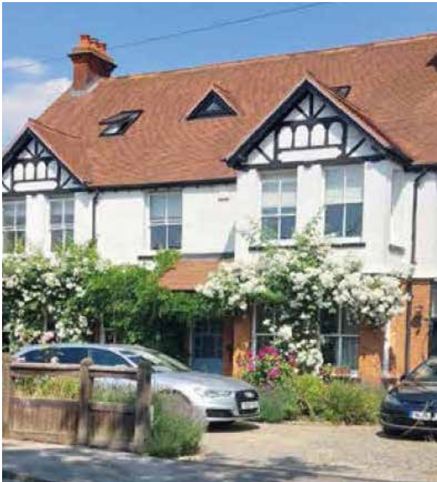
Detached building featuring 2 storey boxed bays and windows with vertical emphasis.
