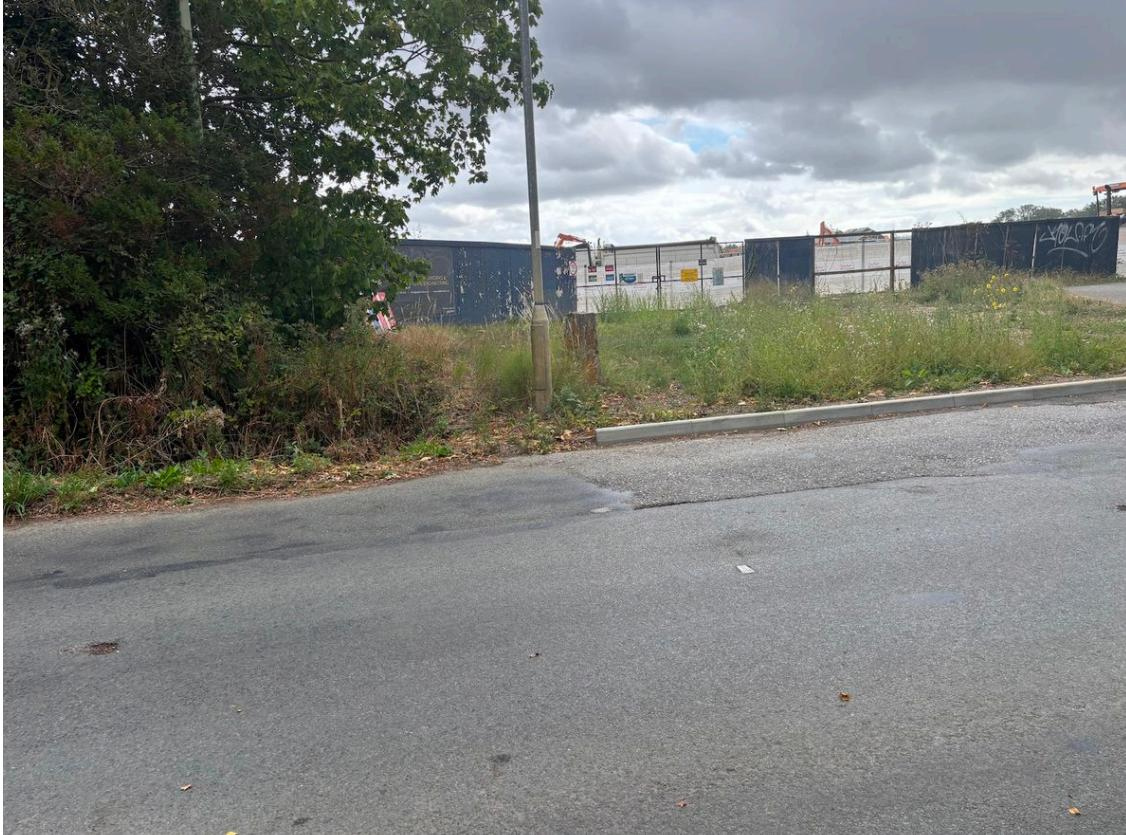
A pedestrian crossing is proposed over the access road. It is not clear to the Audit Team whether hoarding will be installed along the access road. This may cause an obstruction to the pedestrian intervisibility of the crossing. This may result in entering vehicles colliding with pedestrians when they step into the carriageway.
