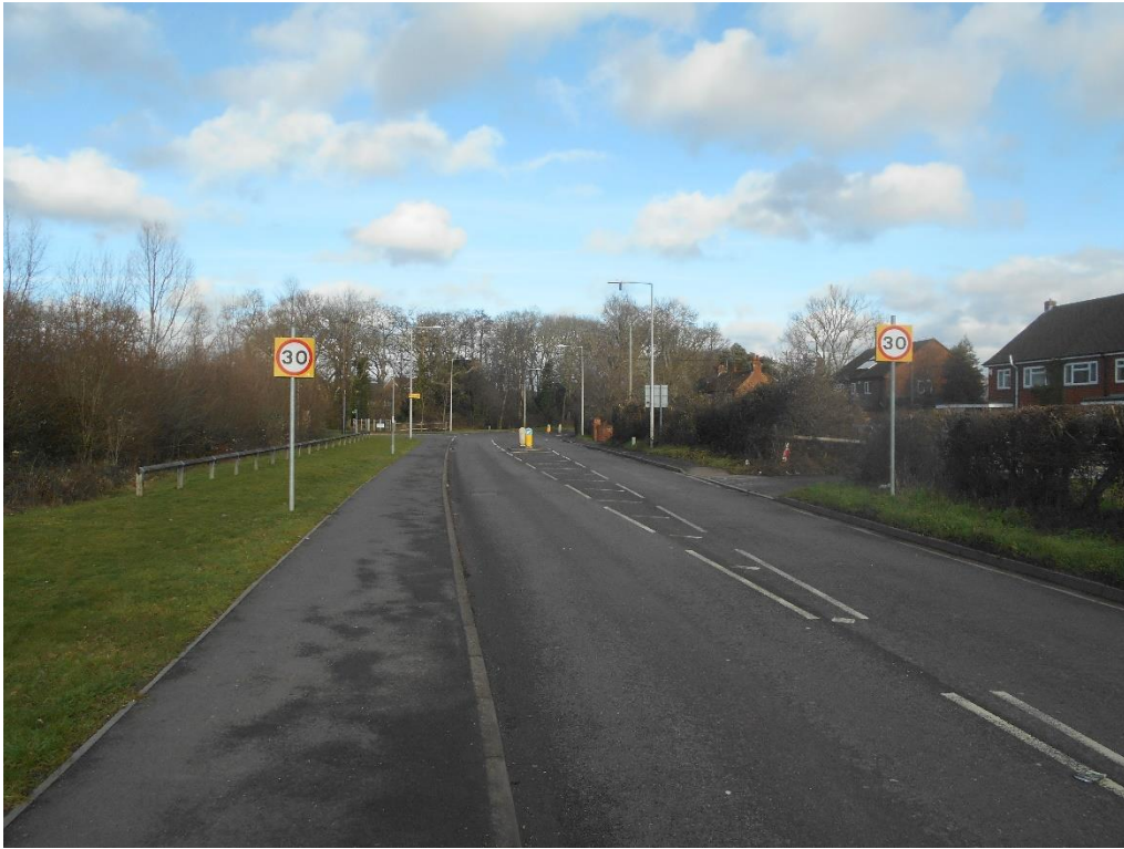
Looking north on Hyde End Road from the site of the proposed Toucan crossing. The path on the left is to be widened to 3.0 metres to accommodate shared use, with a 0.5 metre wide block paved margin
