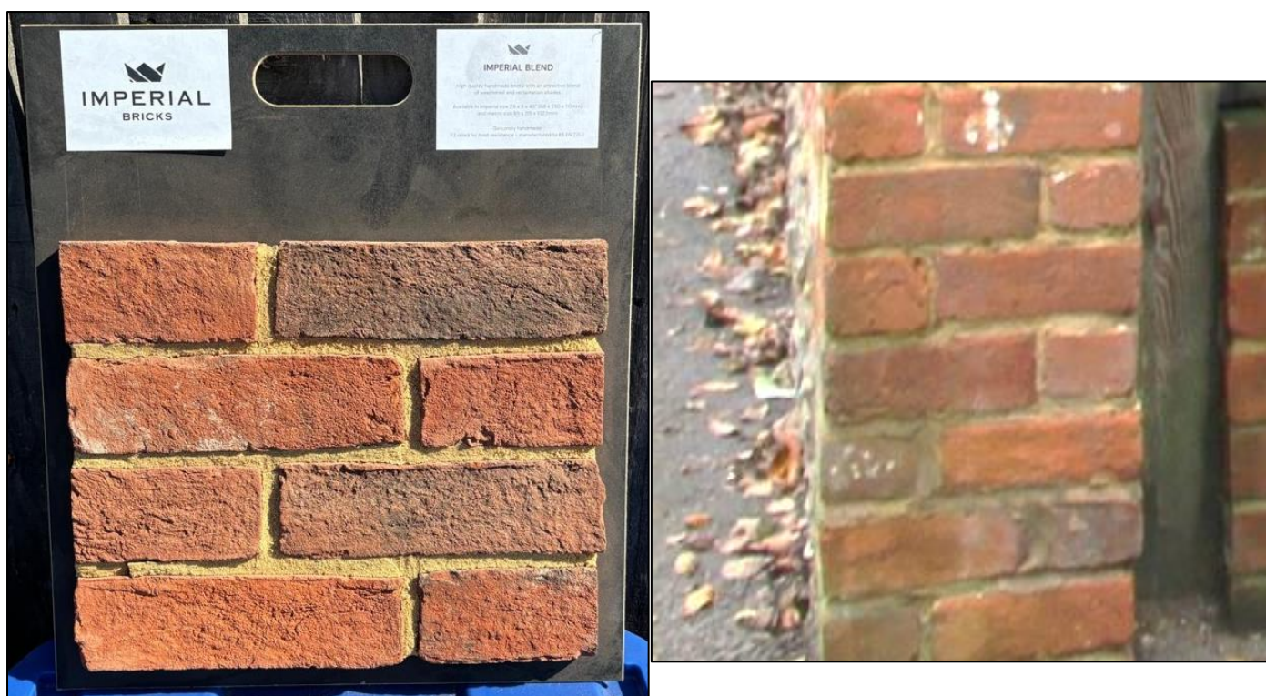
Photograph 2 – Imperial blend brick for external surface of new detached garage and Photograph 3 showing the existing brickwork to the frontage along Station Road
