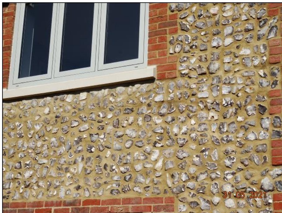
Photograph 4 – Flint faced concrete block to be used in the construction of the detached garage
