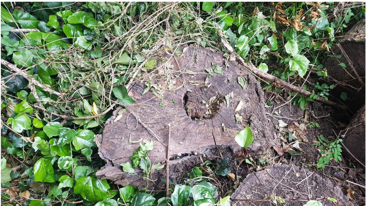
Photo 6 – Cross section of wood from fallen trunk. Note asymmetrical base and central column of decay.
