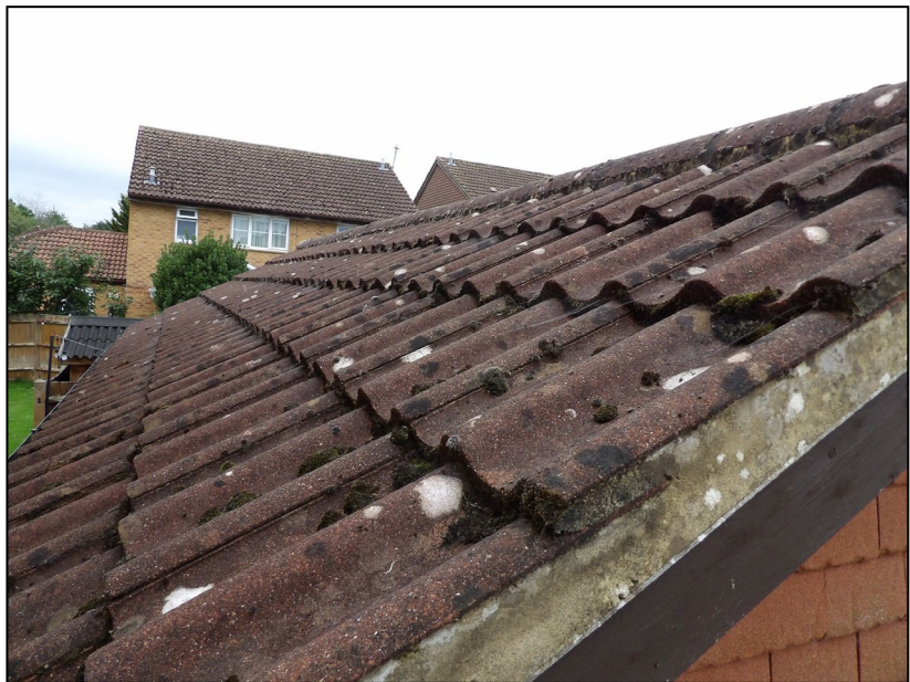
Figure 11. Example of tightly fitted hanging tiles. 52 Poundfield Way, Twyford. 18.09.25
