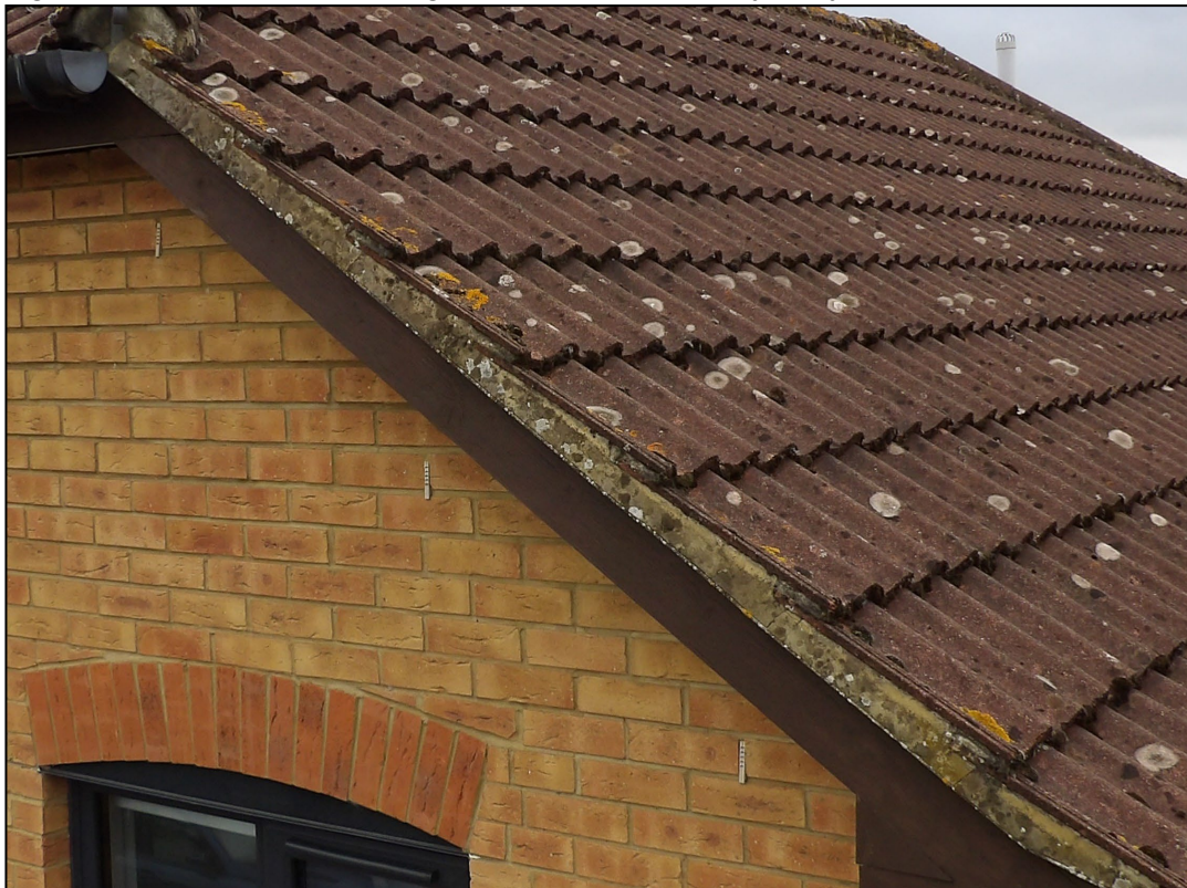
Figure 6. Example sealed verges. 52 Poundfield Way, Twyford. 18.09.25
