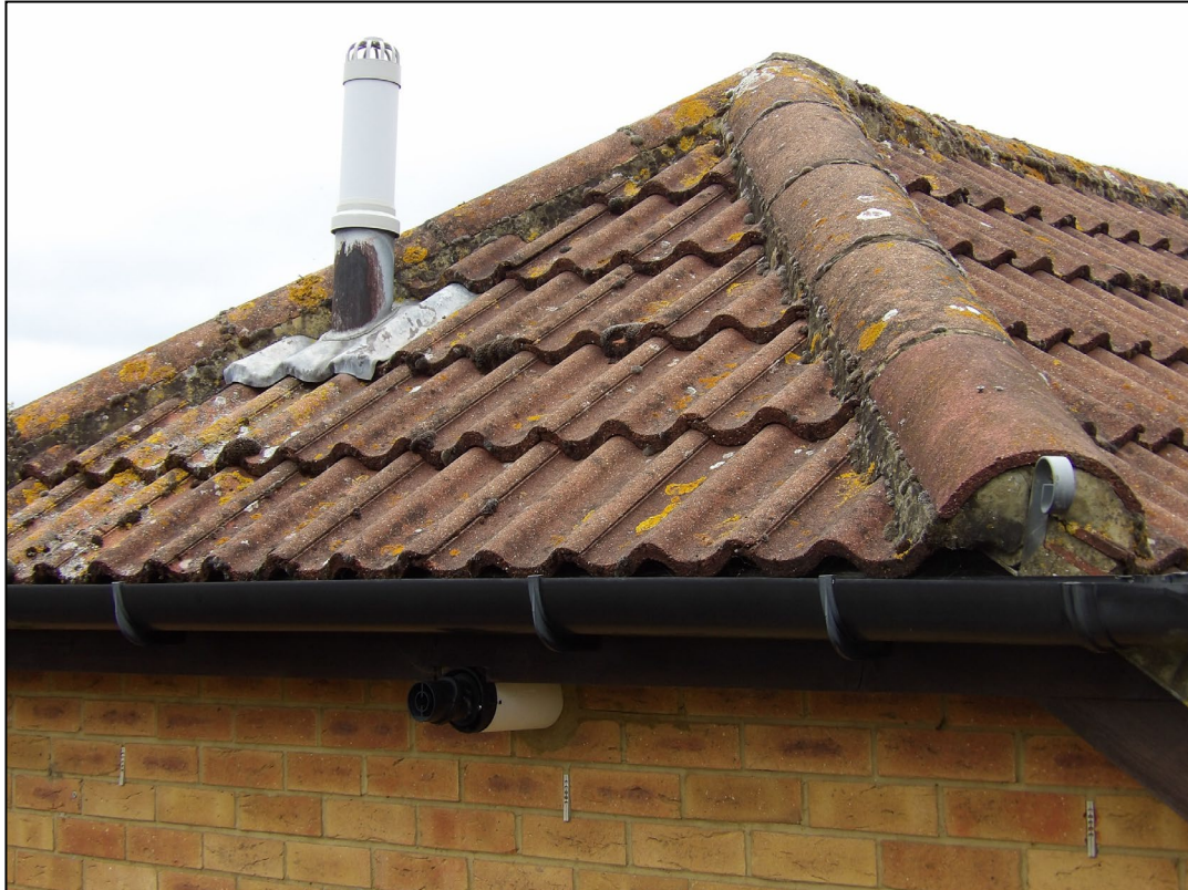
Figure 5. Example of ridge and hip tiles. 52 Poundfield Way, Twyford. 18.09.25
