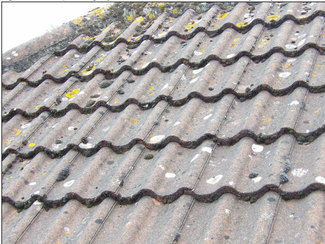
Figure 4. Example of tightly fitted roof tiles. 52 Poundfield Way, Twyford. 18.09.25
