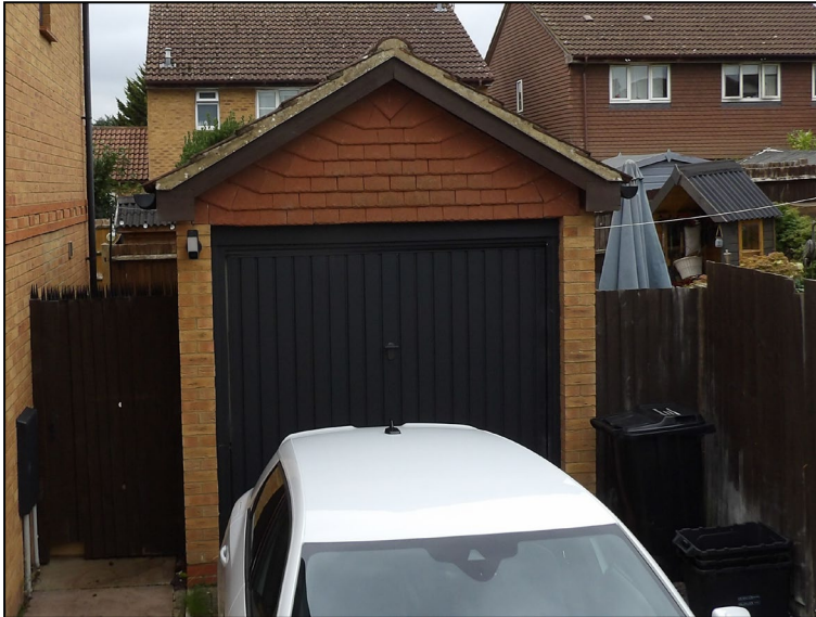
Figure 10. Example sealed roof and ridge tiles on garage. 52 Poundfield Way, Twyford. 18.09.25
