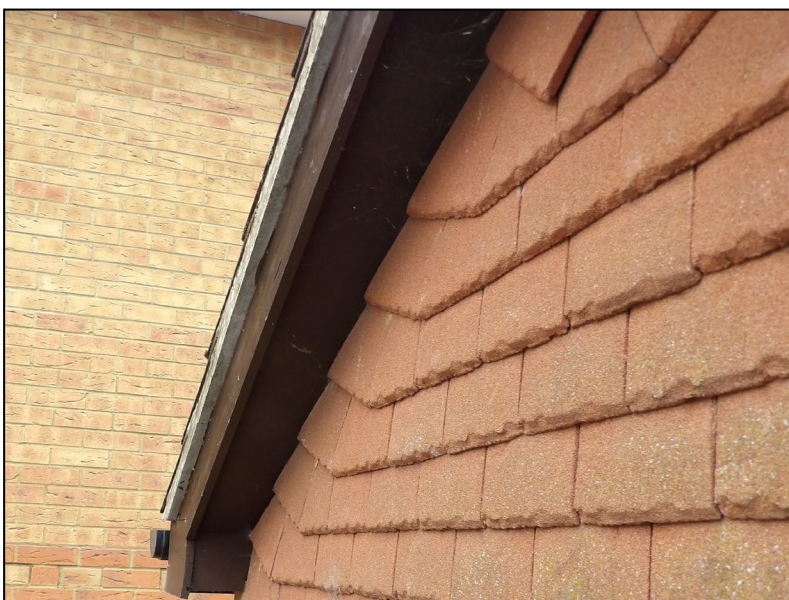
Figure 11. Example of tightly fitted hanging tiles. 52 Poundfield Way, Twyford. 18.09.25
