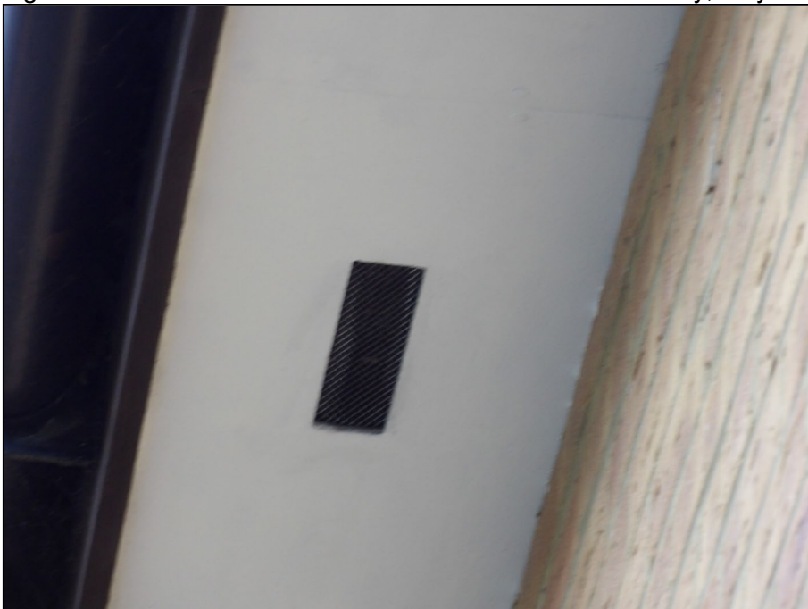
Figure 8. Ventilation holes in soffit boxes. 52 Poundfield Way, Twyford. 18.09.25
