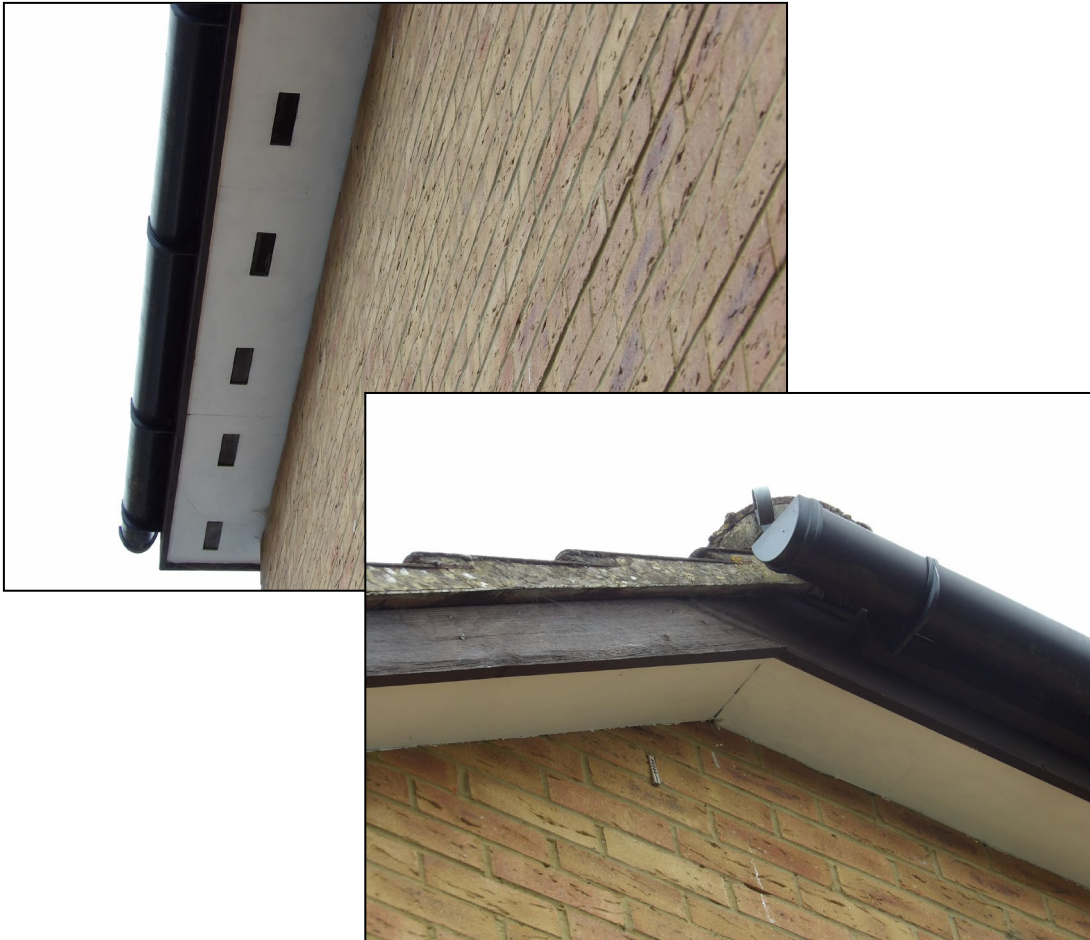
Figure 8. Ventilation holes in soffit boxes. 52 Poundfield Way, Twyford. 18.09.25
