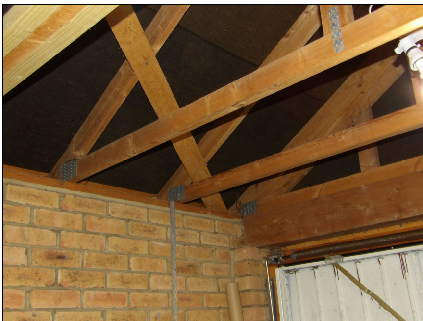
Figure 13. Internal view of garage roof. 52 Poundfield Way, Twyford. 18.09.25
