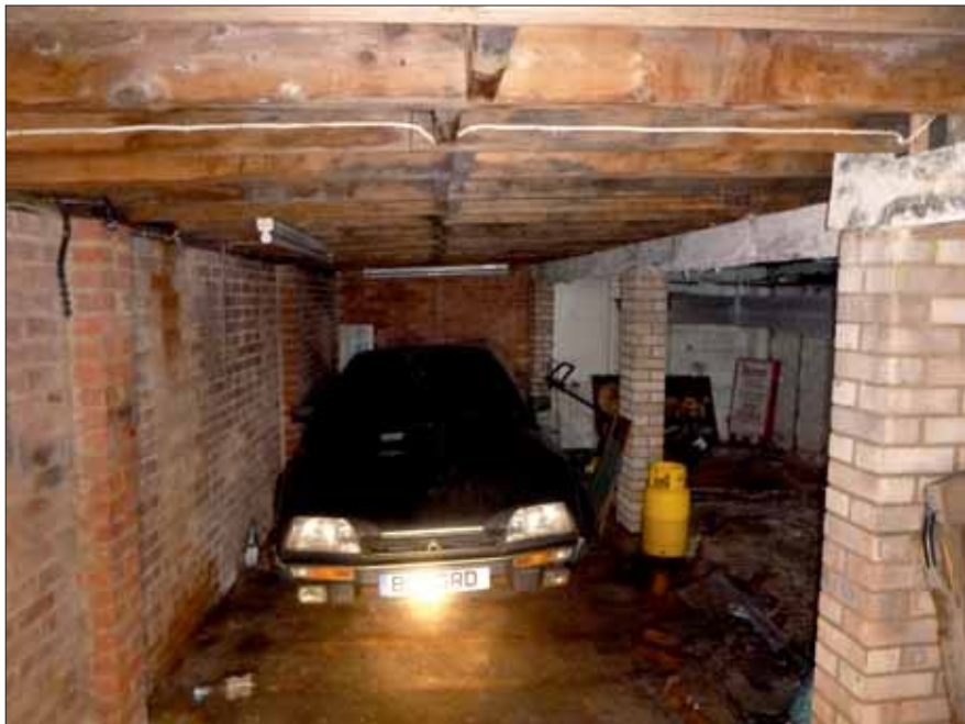
Photograph 3: Showing the interior of the workshop, with an unlined roof.
