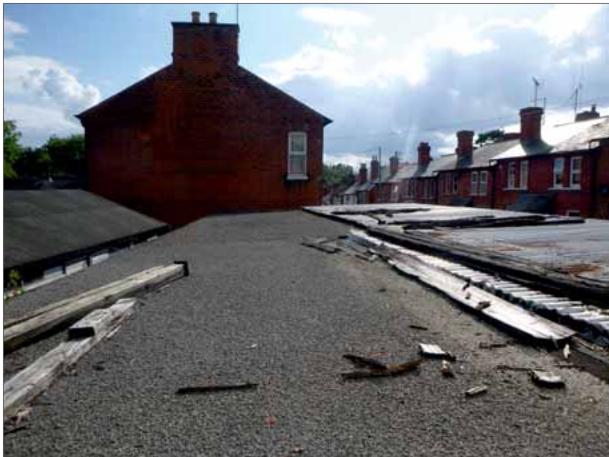
Photograph 4: Showing the flat roof of the workshop.
