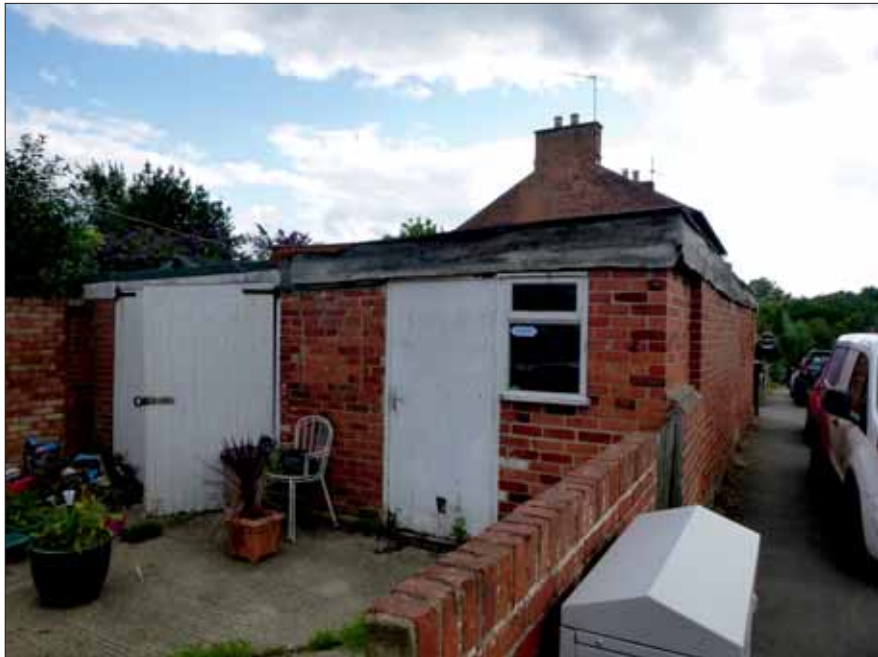
Photograph 1: Showing the front and side elevations of the workshop.
