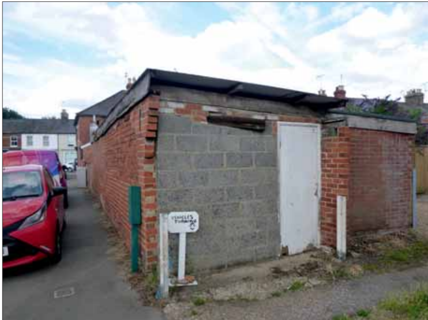
Photograph 2: Showing the rear elevation of the workshop.
