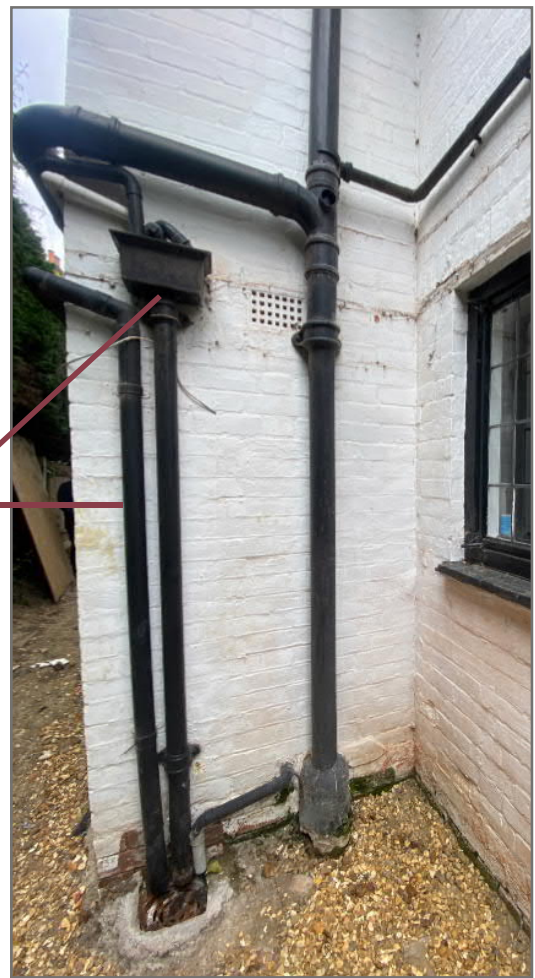
Image 07: View of south elevation of west gable return
