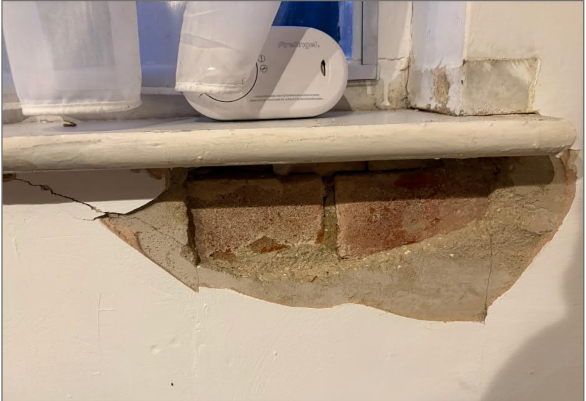
Image 18: Exposed brickwork to the First Floor Master Bedroom: proposed to infilled with lime plaster
