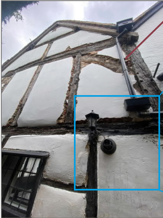
Image 05a: View of West gable
