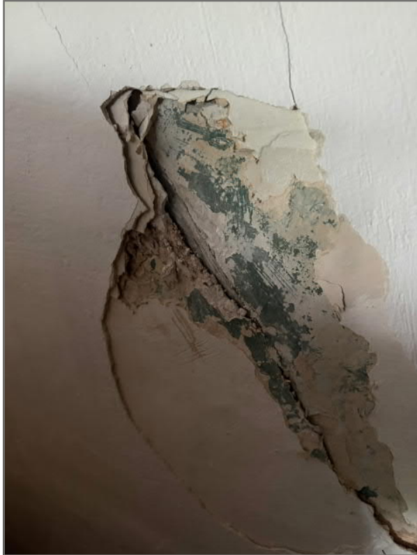
Image 20: Example of wall condition where the proposal is to strip wallpaper where historic lime plaster exists and repair historic lime plaster on a like-for-like basis.
