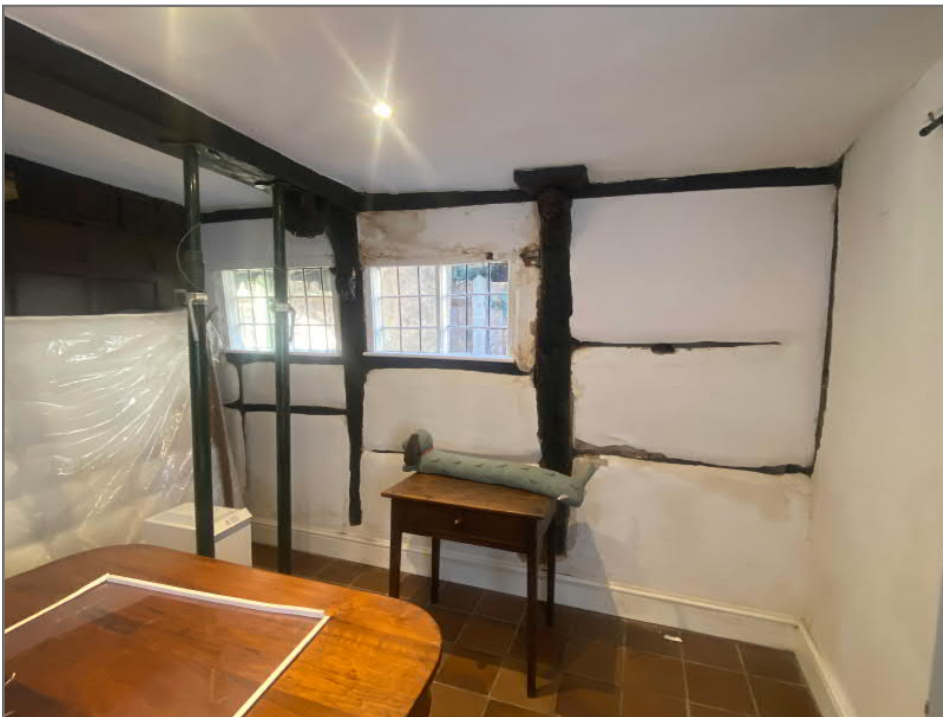
Image 13: Exposed internal timber construction to the Ground Floor West gable: proposal to remove all modern impervious paints and varnish to all historic timbers using soda blasting
