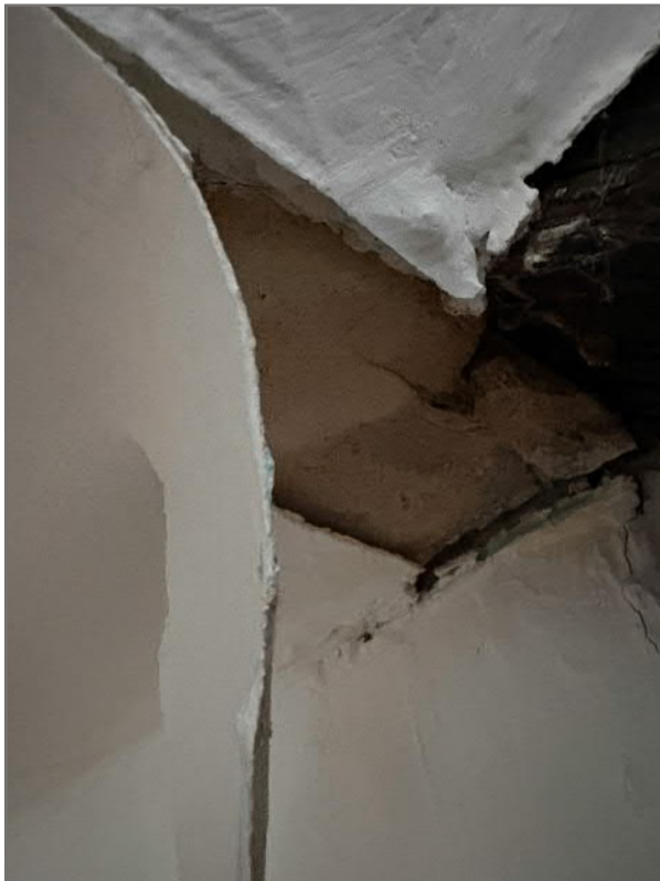
Image 21: Proposal to remove of cement and gypsum materials and replace with a vapour-permeable build-up, or split laths, as appropriate, ready for lime plastering.
