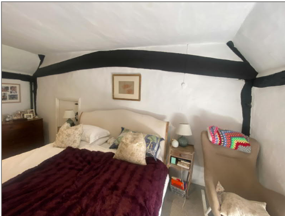
Image 17: Exposed internal timber construction to the First Floor Master Bedroom: proposal to remove all modern impervious paints and varnish to all historic timbers using soda blasting
