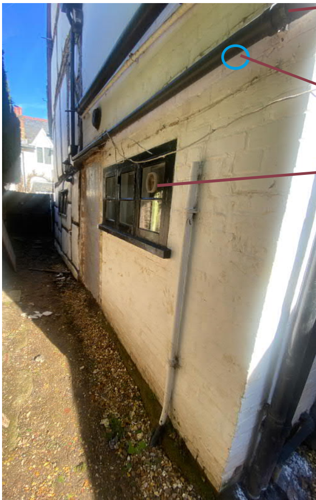
Image 06: View of south elevation of west gable return
