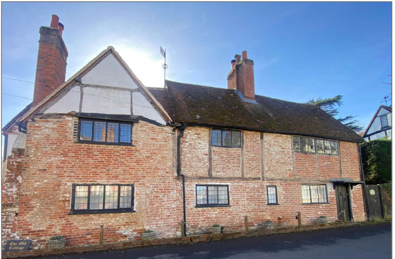
Image 03: View of North elevation along Pearson Road
