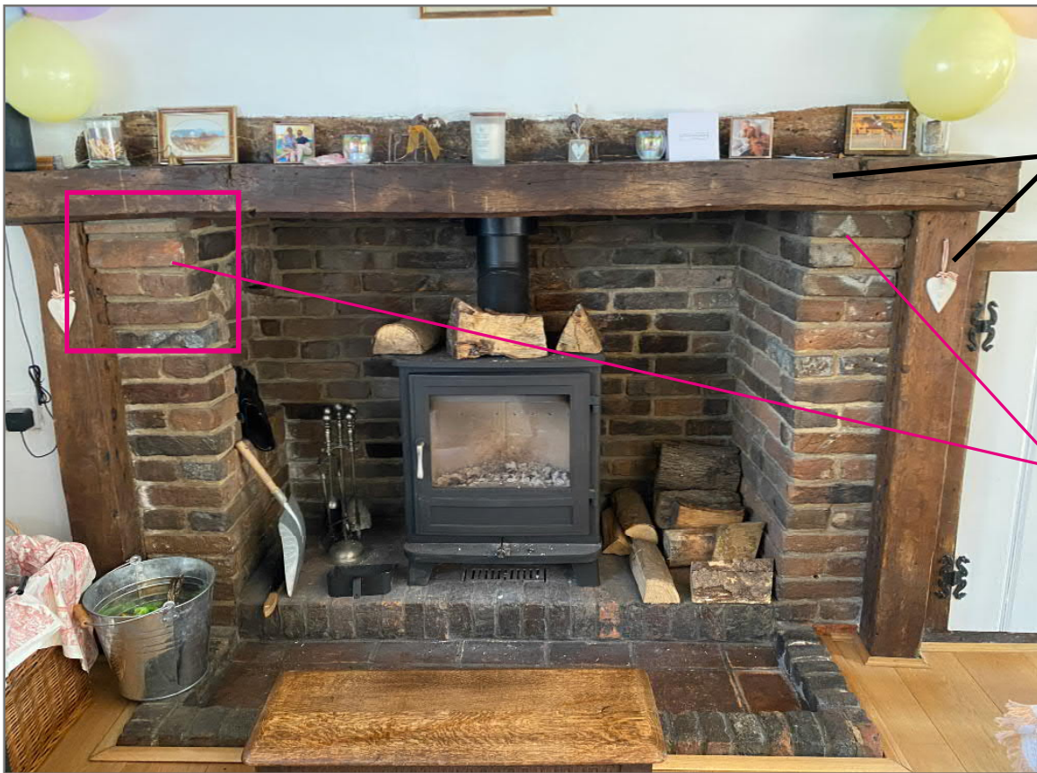
Image 12a: Existing fireplace to Ground Floor (East Wing) with modern brickwork and lintel
