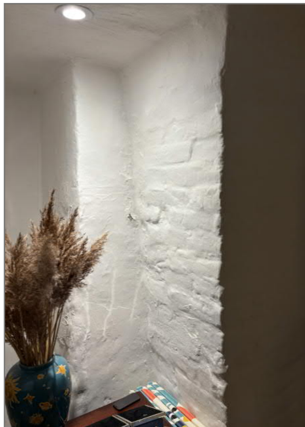
Image 19: Example of area proposed for masonry cleaning
