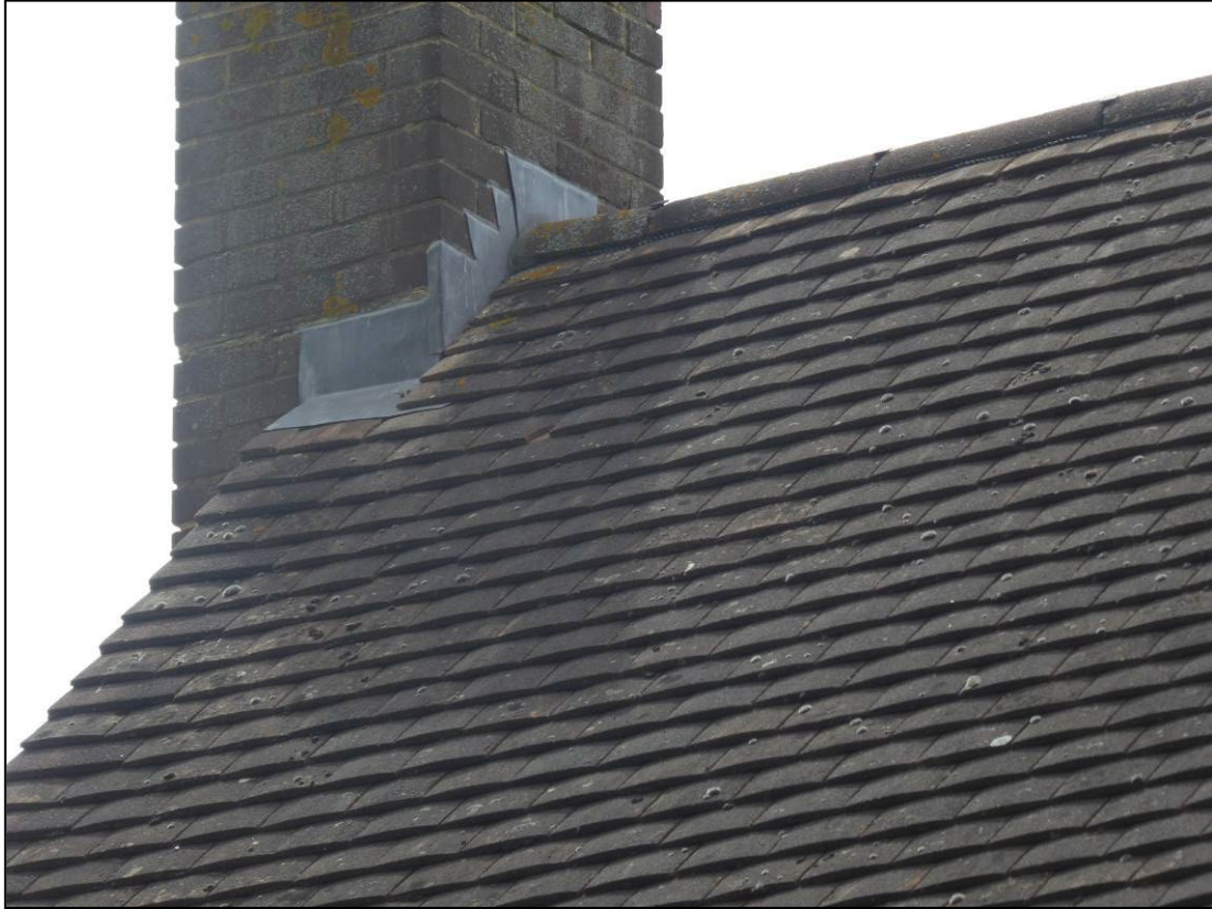
Figure 7. Lead flashing around chimney. 8 Salmond Road, Shinfield, 16.07.24
