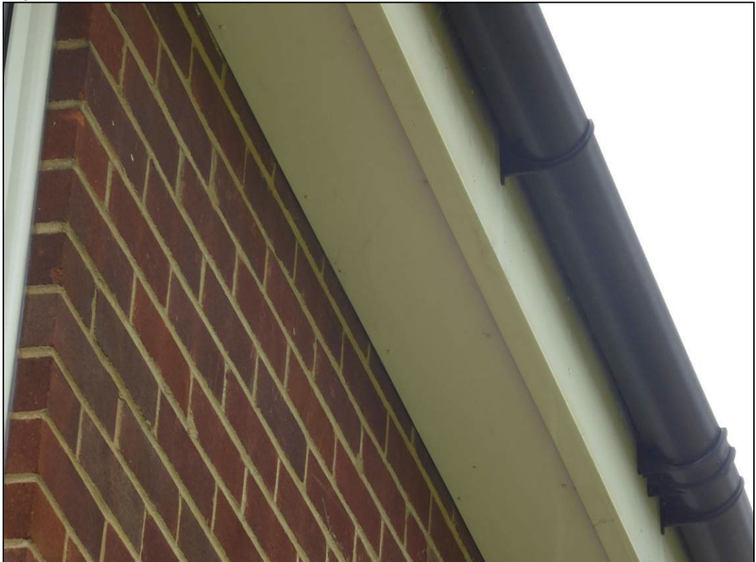
Figure 8. Soffits and fascias. 8 Salmond Road, Shinfield, 16.07.24
