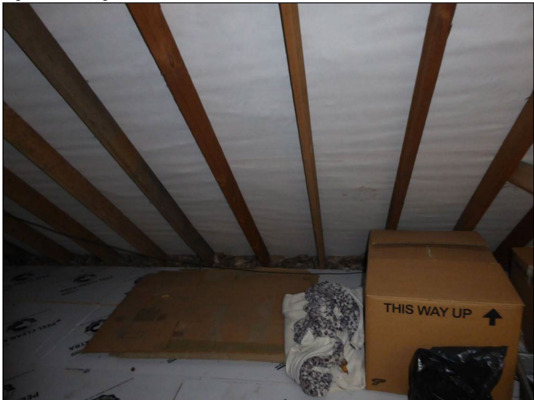
Figure 13. Lining of roof tiles in loft. 8 Salmond Road, Shinfield, 16.07.24
