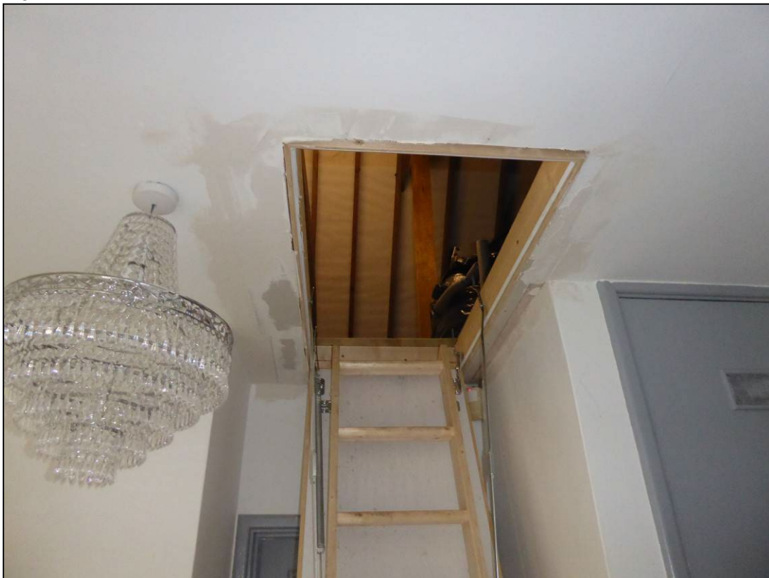
Figure 11. Example of loft hatch. 8 Salmond Road, Shinfield, 16.07.24
