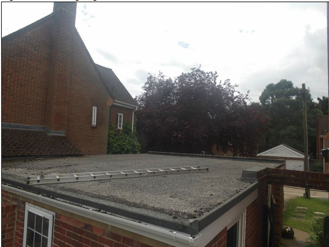
Figure 10. Roof of garage. 8 Salmond Road, Shinfield, 16.07.24
