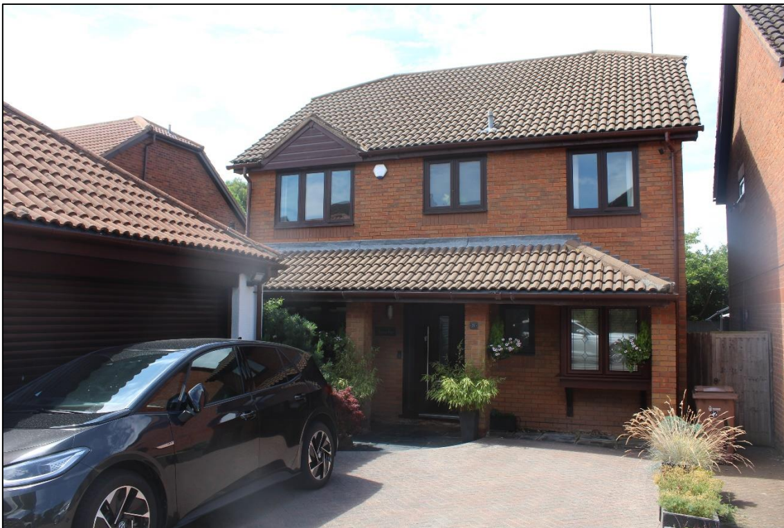
Photograph 1 – Front elevation as viewed from Thorn Close
