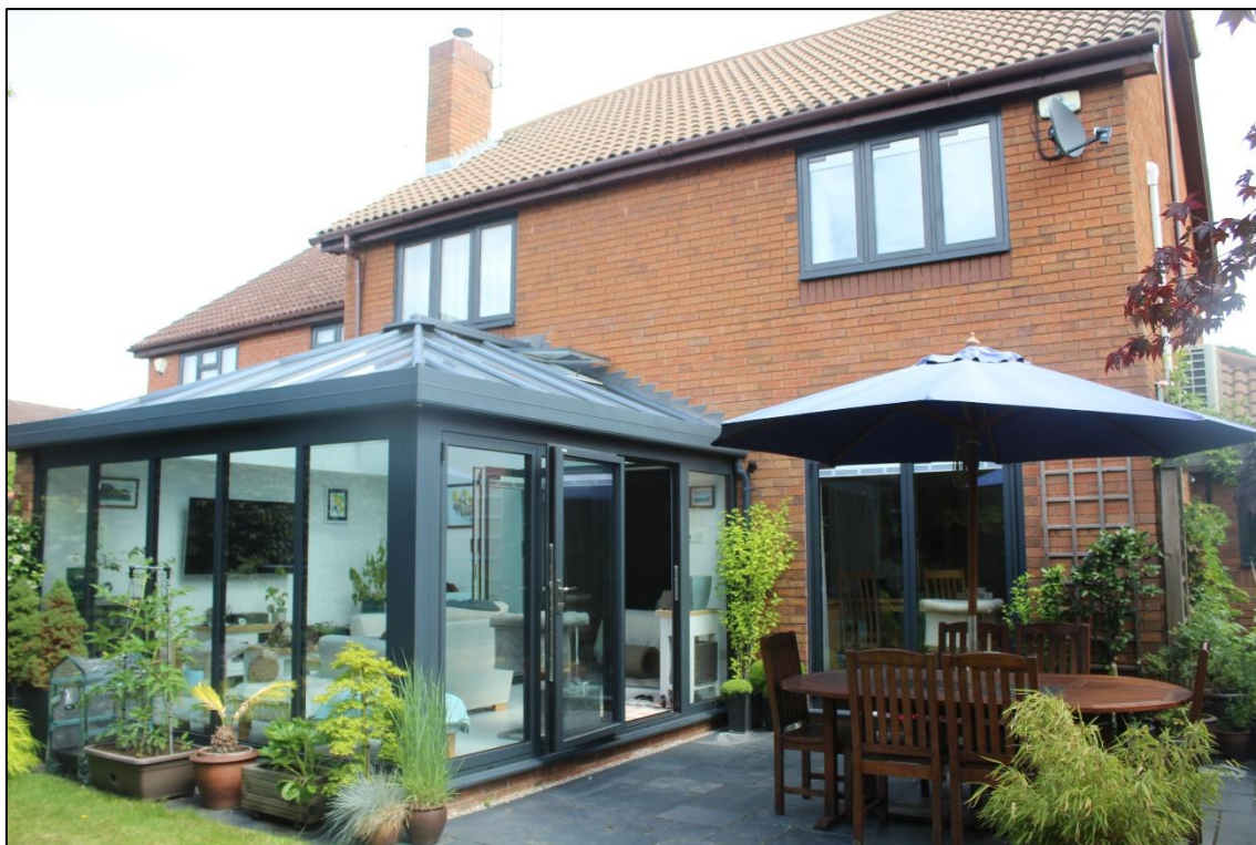
Photograph 2 – Existing conservatory as viewed from the rear garden
